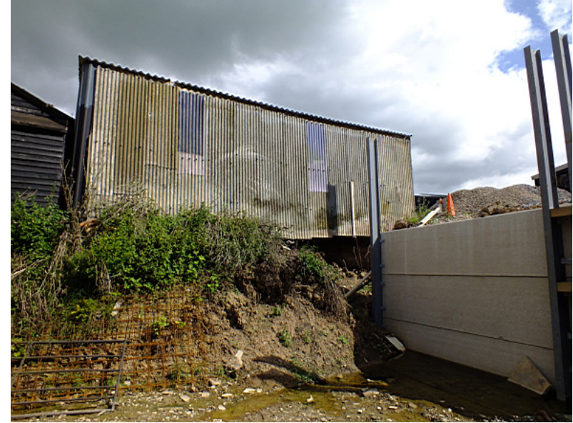
Photo 6: Construction of the retaining wall has allowed slumping of soil from under the shed leaving its floor unsafe.
