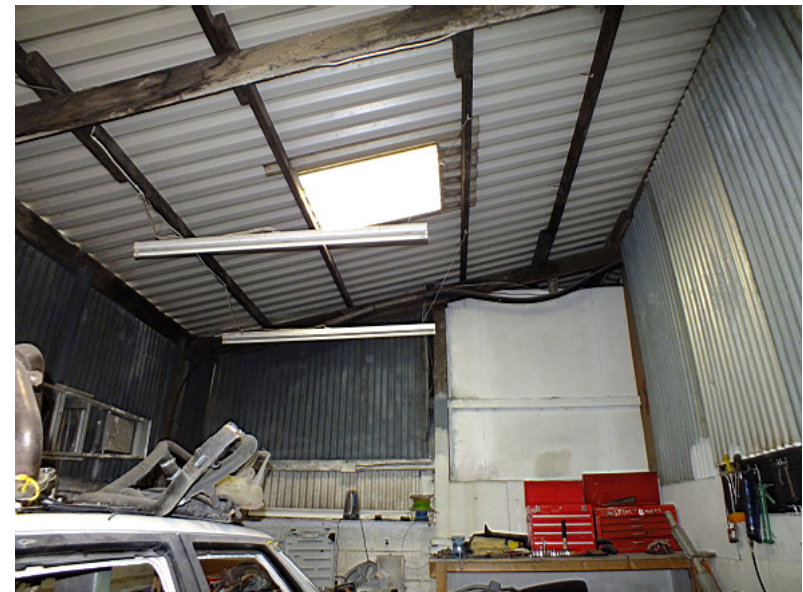
Photo 4: Section d interior showing single skin walls and roof. The void above the white wall of section c was inspected from section a.
