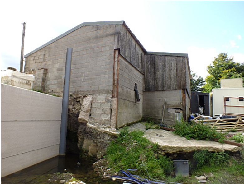
Photo 1: Asbestos 'cladding' on the upper half of the W-facing walls is single-skinned with no voids behind. No bat droppings were found on the ground underneath.
