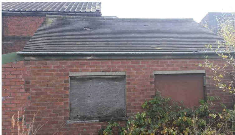
Image 16: B9 – western elevation – showing gaps in roof and boarded windows with gaps
