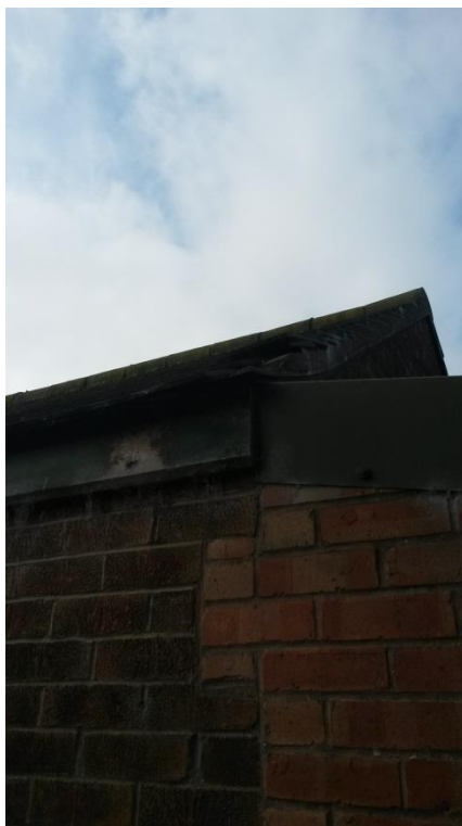
Image 12: B9 – lifted tiles & missing mortar at northern gable end
