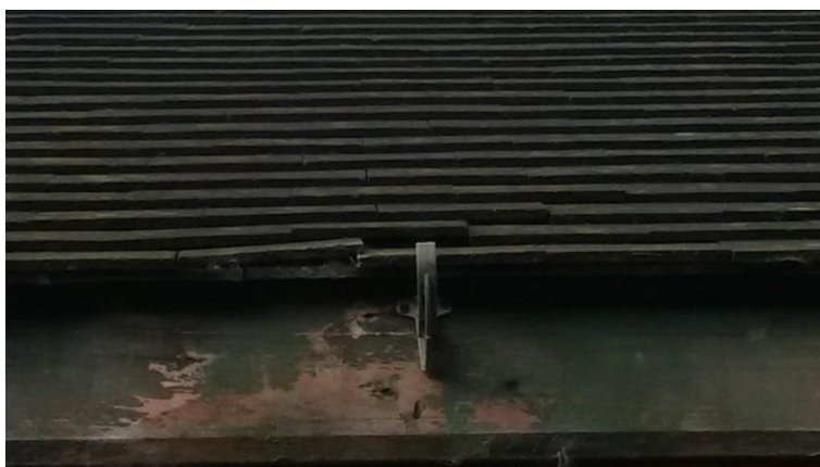
Image 14: B9 – Gaps at eaves on eastern side of roof
