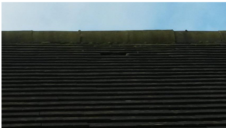
Image 13: B9 – missing tile on eastern side of roof
