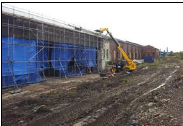
PHOTO 8 Concrete asbestos removal
