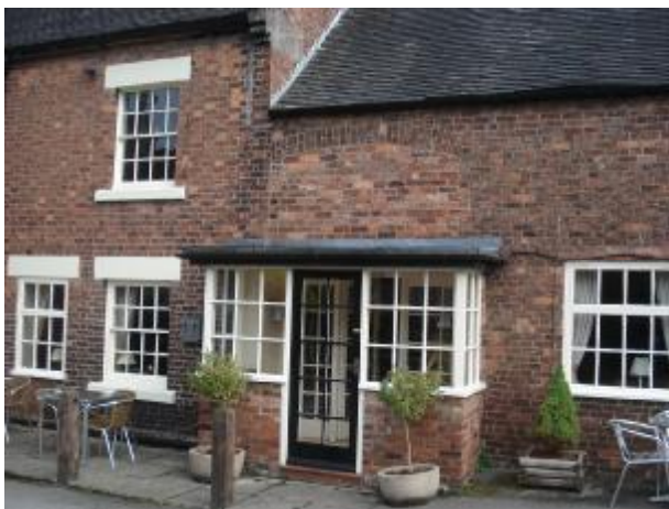
Existing side entrance lobby - a 21 st Century addition.
