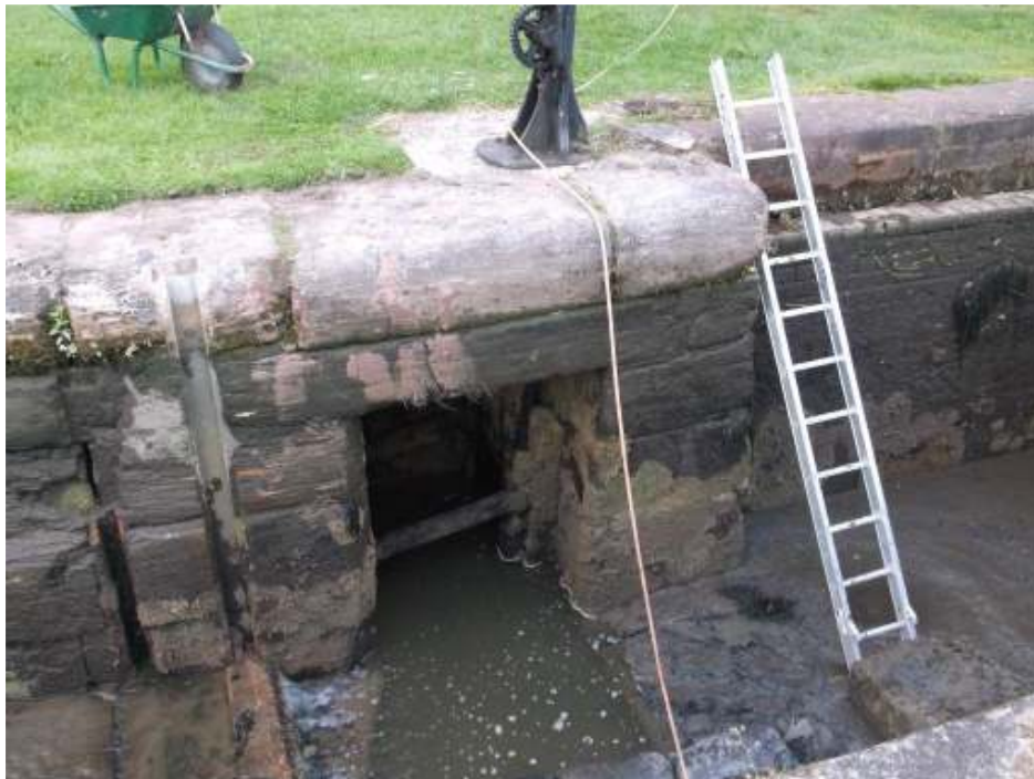
Photo of dewatered Paddle Chamber 1.
