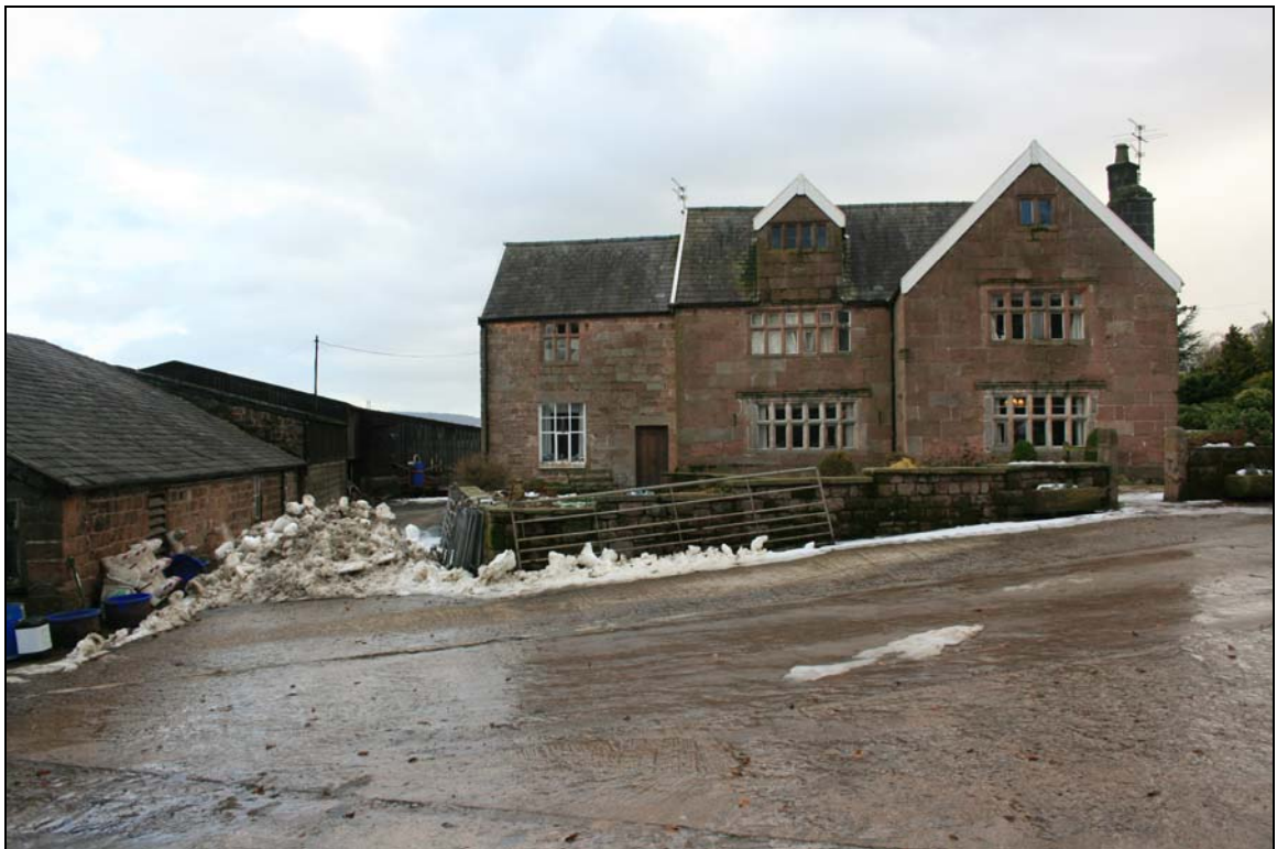
1. Cloud House Farm and its outbuildings, looking southeast
