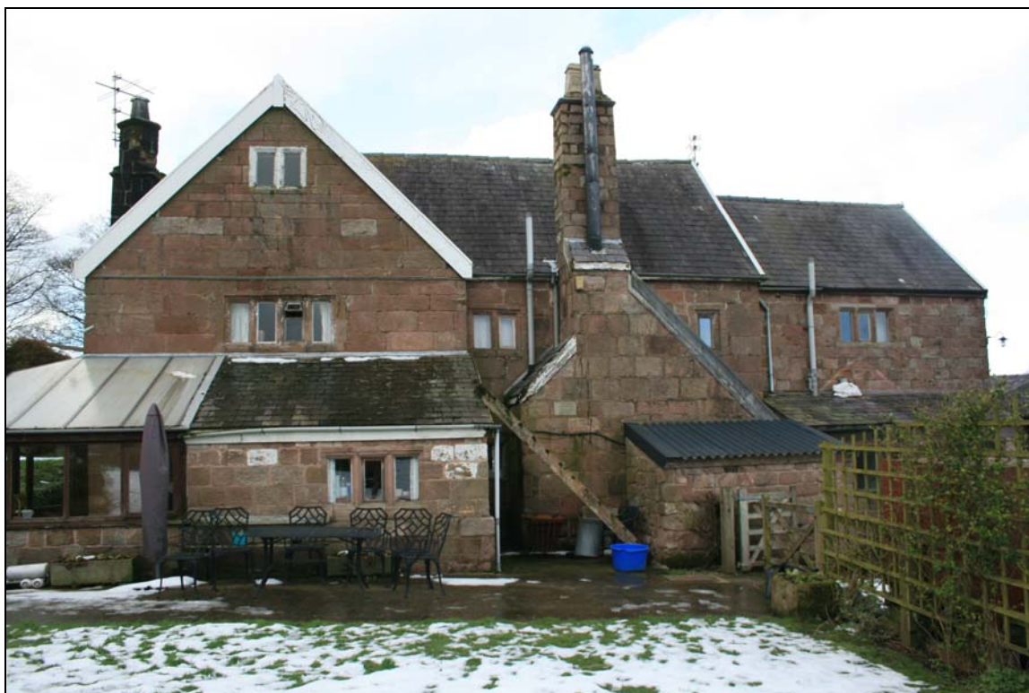
4. Rear showing single-storey 20 th century additions
