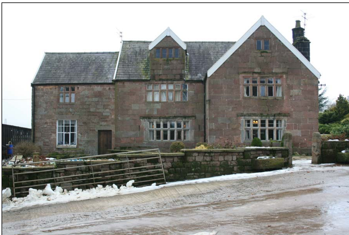
3. The principal (northwest-facing) elevation of Cloud House Farm, showing the central housebody range, crosswing wing on right and service wing on left
