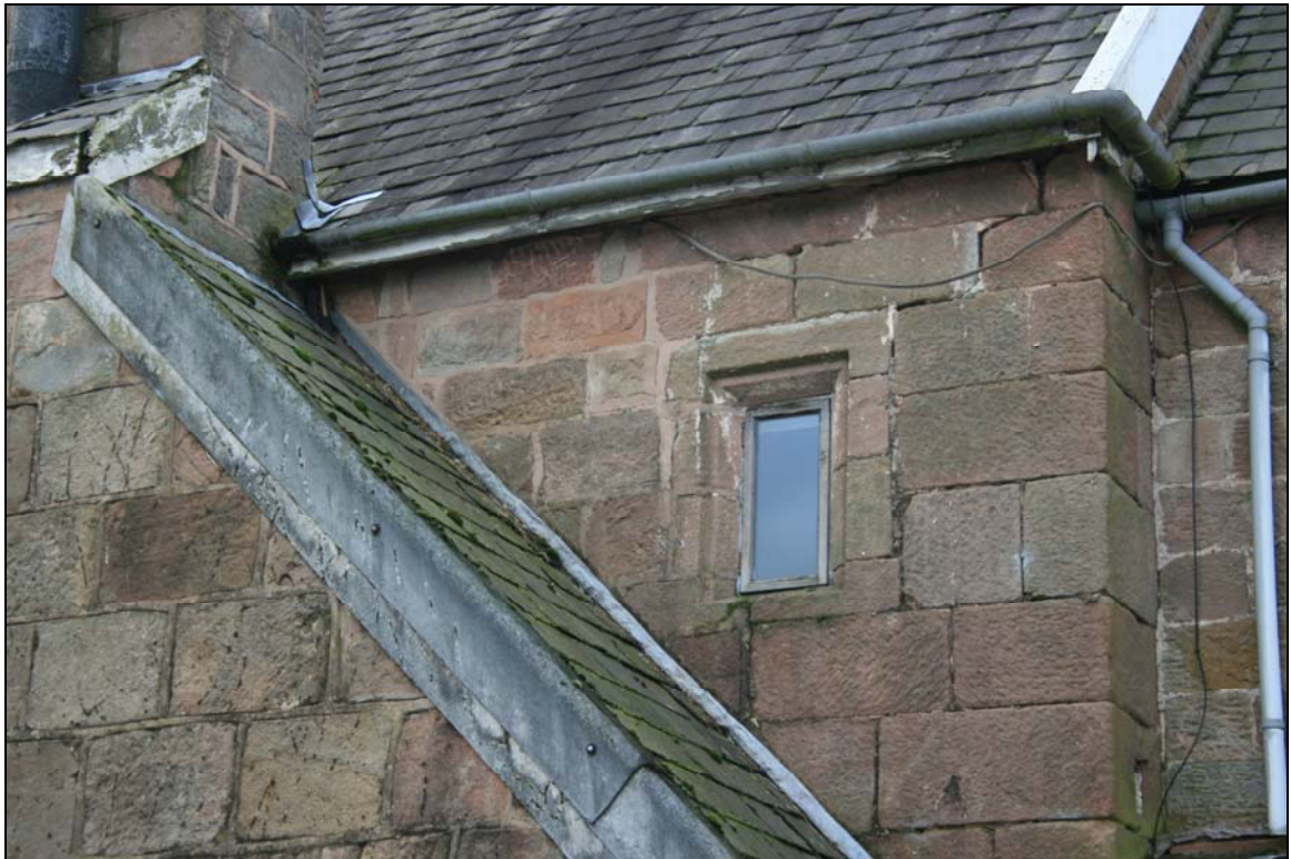
14. First floor rear window: widening is proposed to the left
