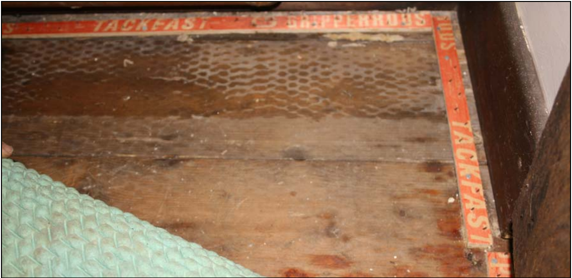
16. Example of section of probably 20 th century boards on first floor
