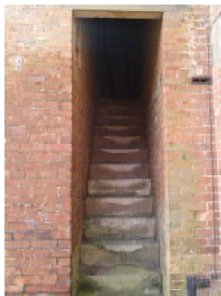
Plate 6: Open stairwell & Air vent
