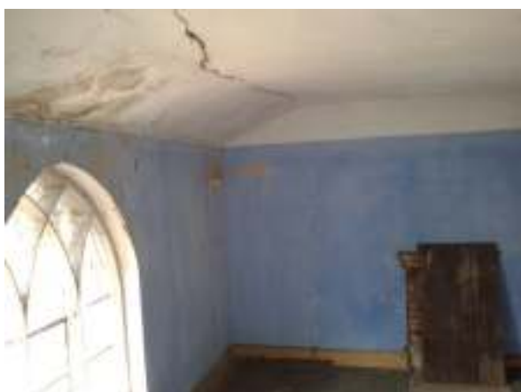
Plate 3: Building B Interior
