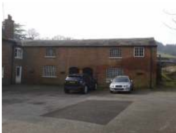
Plate 2: Building A Exterior
