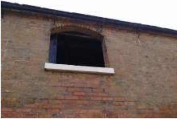
Plate 7: Window with shuttering providing access for bats
