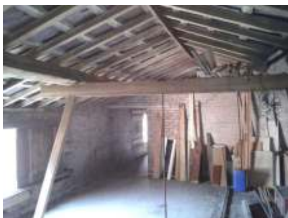
Plate 4: Building B Interior
