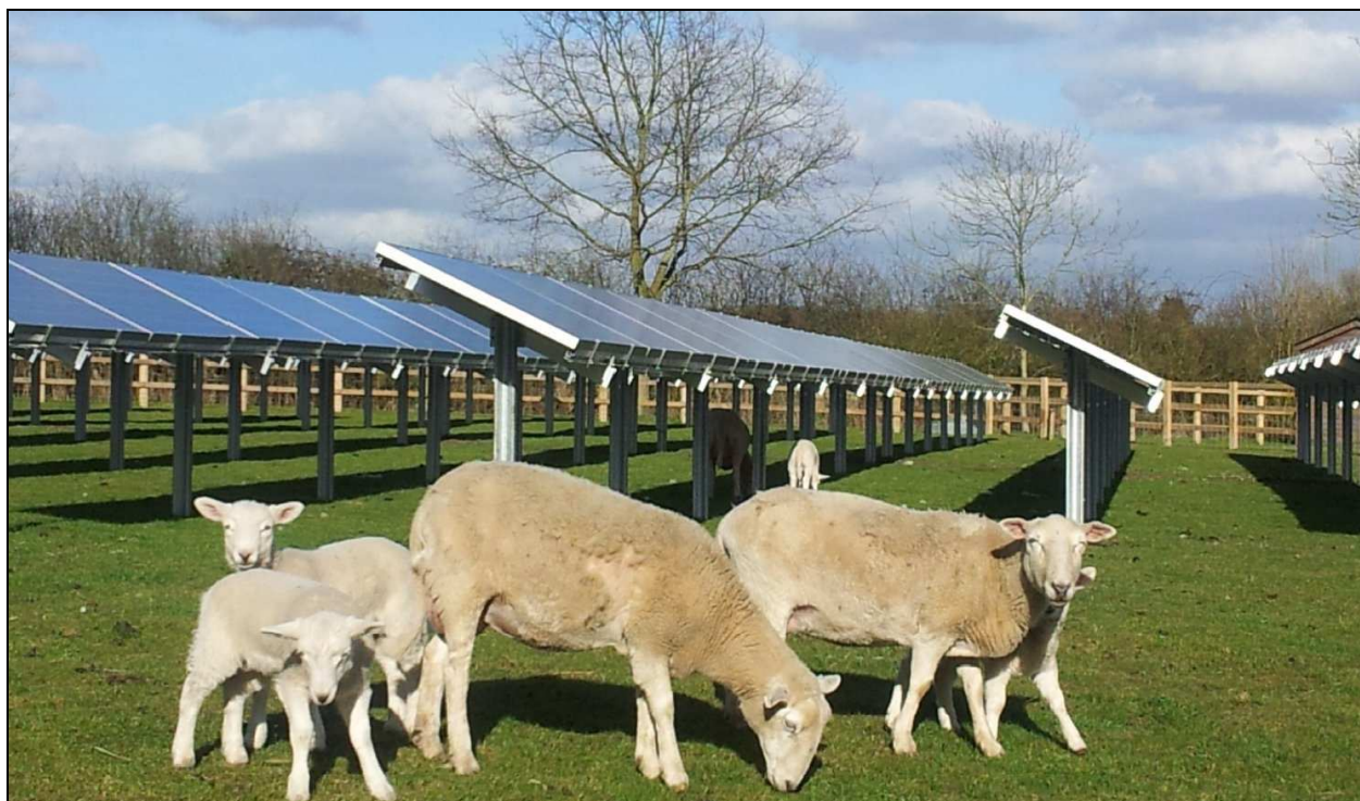
Figure 9 Solar panels of the type proposed at Lower Newton Farm
