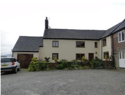
Fig 14. Existing Farm House
