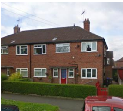
Fig 13. Local Brick Housing
