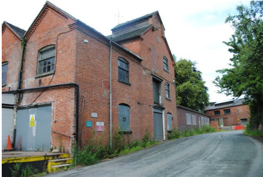
Photograph No. 3: View on North Elevation of East and West Buildings
