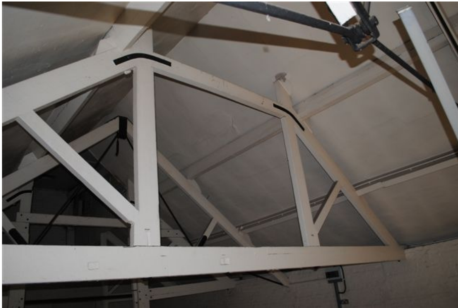
Photograph No. 14: Part View of Roof Truss to West Building
