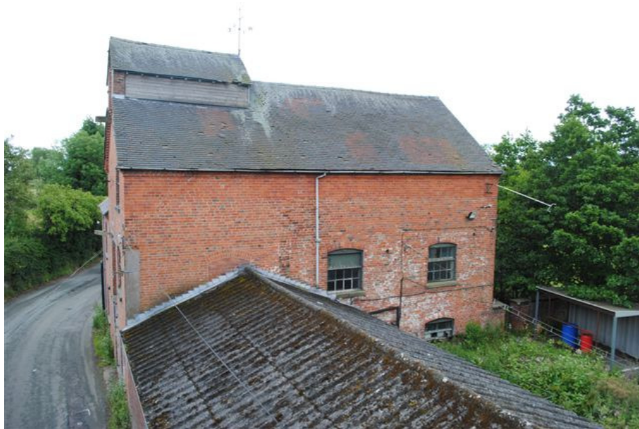
Photograph No. 4: View on West Elevation and Roof of West Building (Note change in brickwork below eaves) (Note canteen building roof in the foreground)
