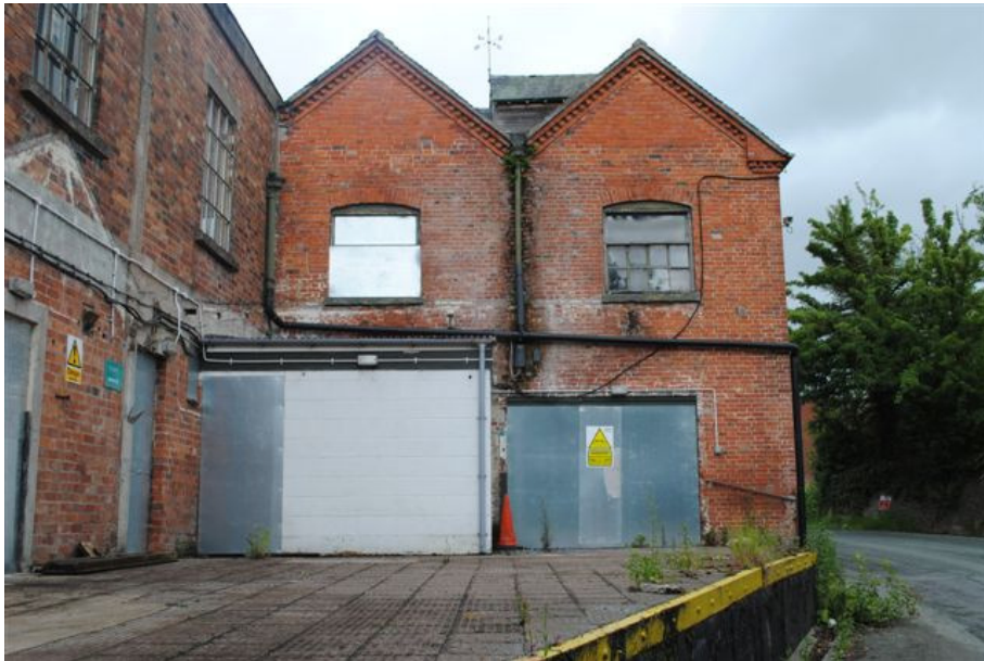
Photograph No. 2: View on East Elevation of East Building
