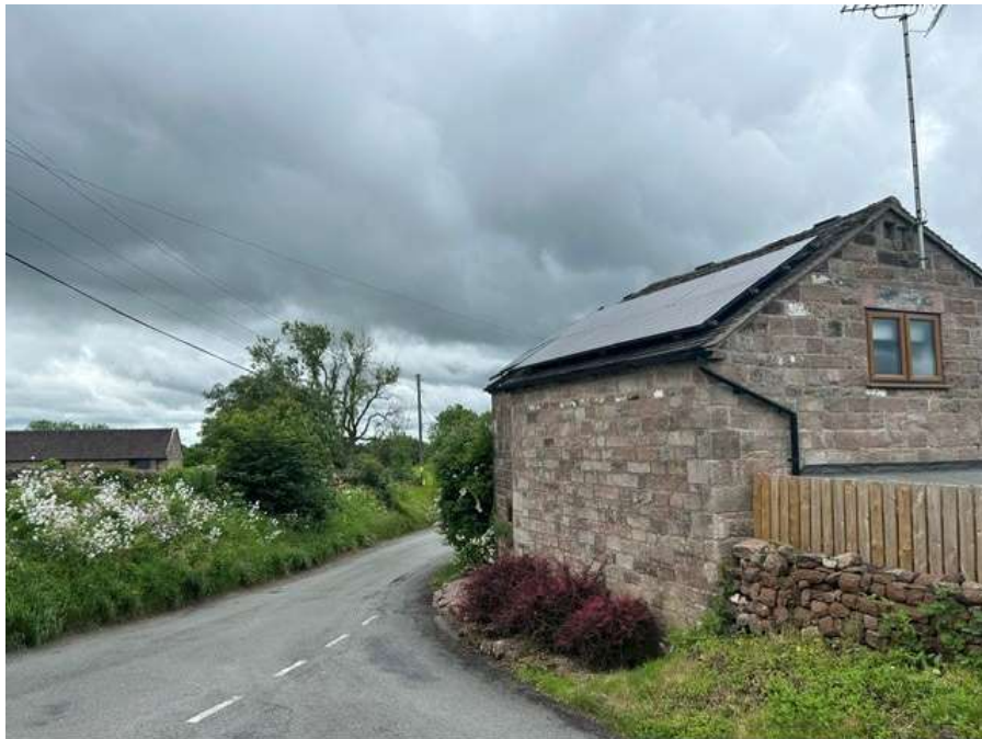
Figure 1: Solar Panels at The Malthouse, Foxt Road.
