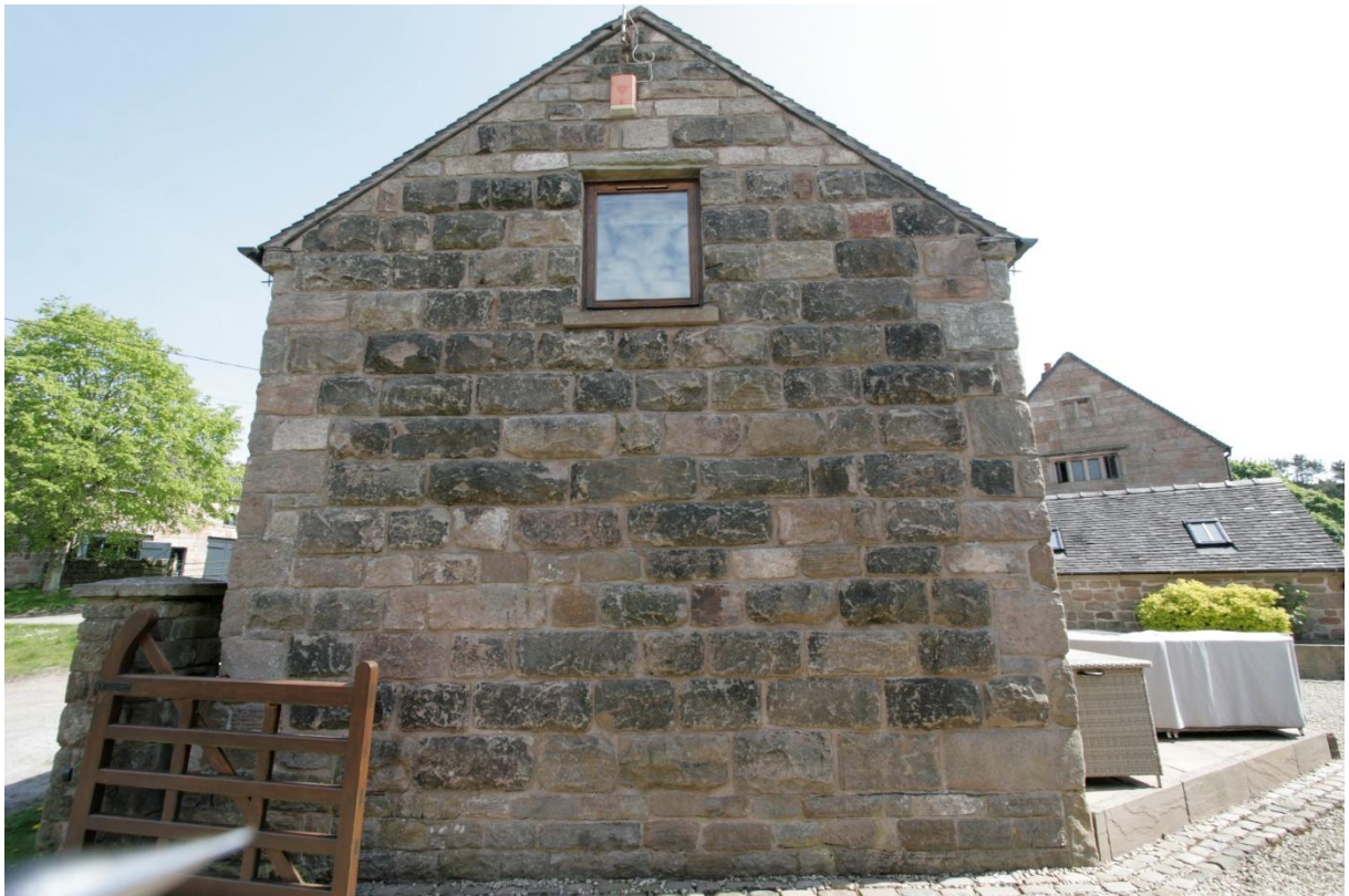
West elevation of The Grange barn previously converted to a dwelling. Window:- ff bedroom 1.
