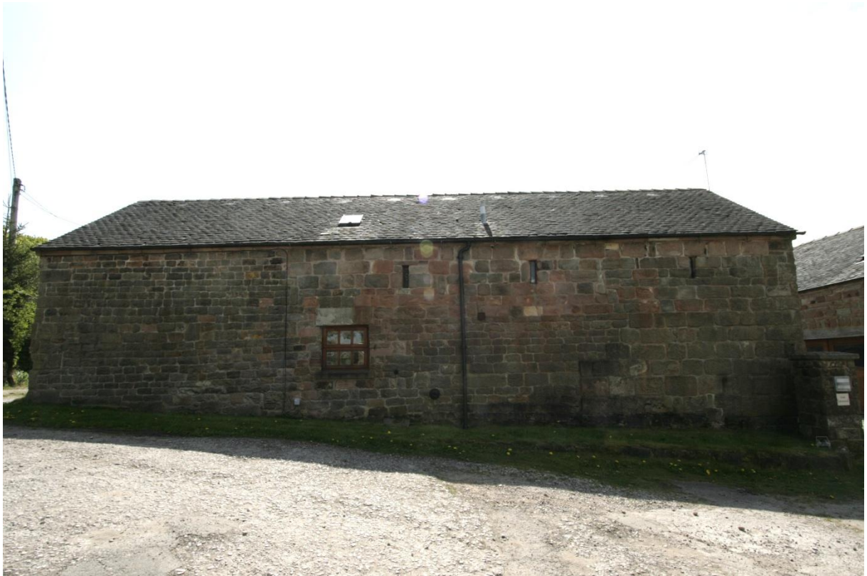
North elevation of The Grange barn previously converted to a dwelling. Window:- gf entrance hall.
