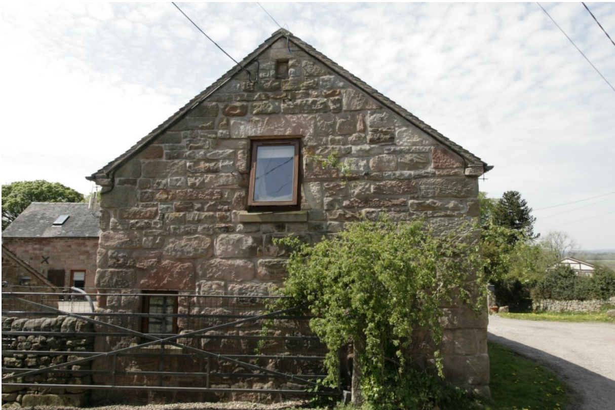
East elevation of The Grange barn previously converted to a dwelling. Windows from left to right:- gf kitchen, ff bedroom 2.
