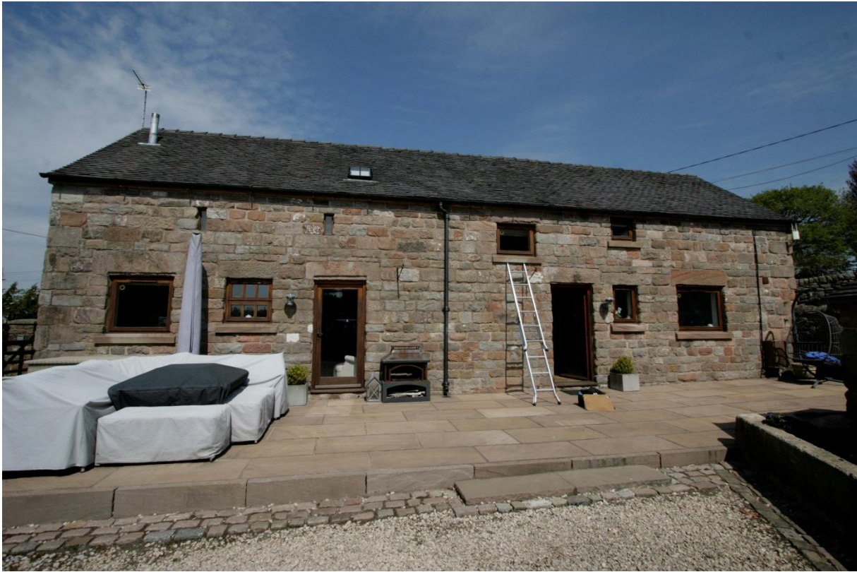
South elevation of The Grange barn, previously converted to a dwelling. Windows from left to right:- gf lounge, gf lounge, door lounge (to be retained), ff stairs, door entrance hall (to be retained), ff bedroom 2, gf kitchen, gf kitchen.
