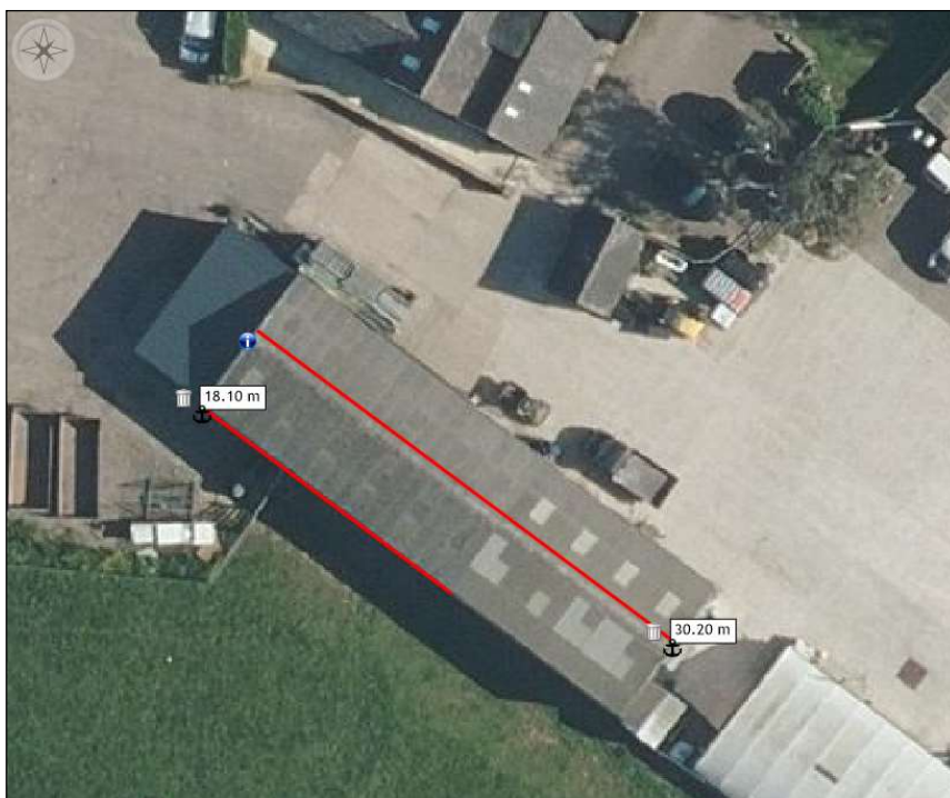
Fig. 3 – The measurement of 30m represents the building subject of this notice. The 18m relates to element B1 (separately subject to a notice by letter dated 31 st July 2016).
