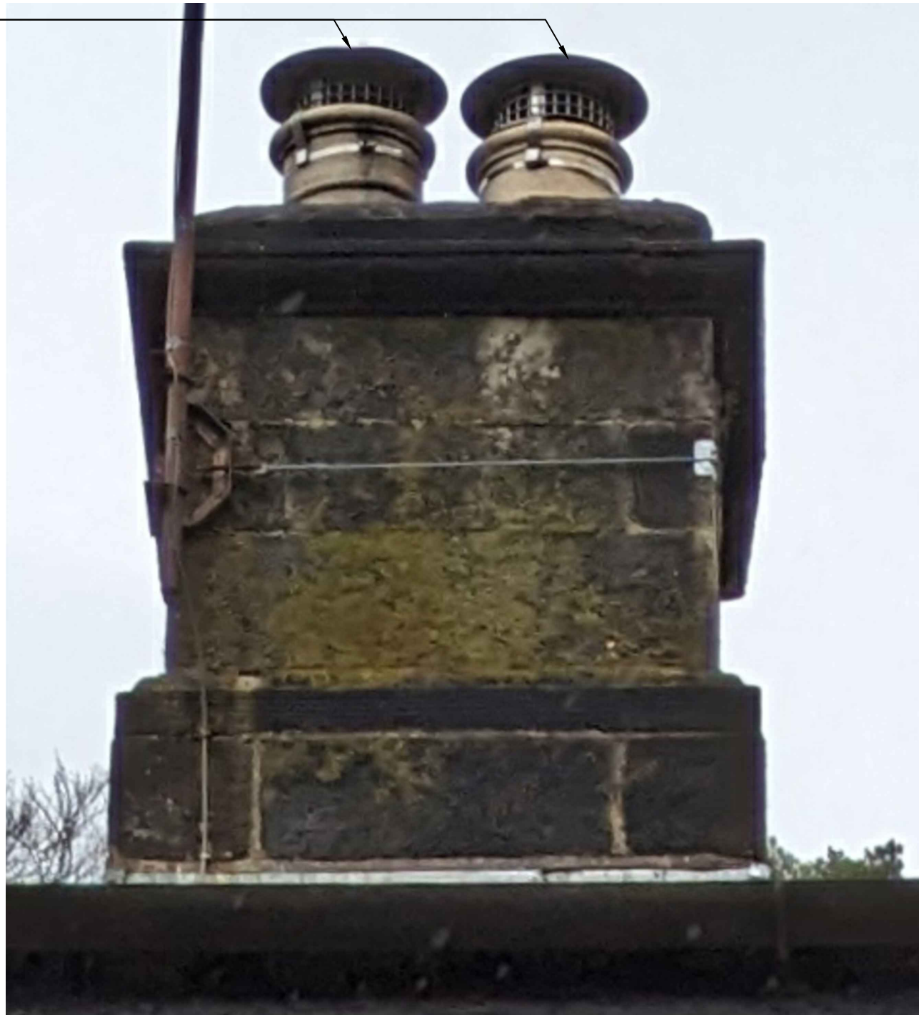
04 3303 Existing Birdguards to Chimney Pots 02 & 03 NTS
