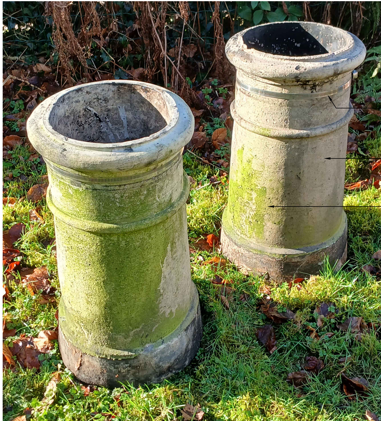
03 3303 Existing Chimney Pots 02 & 03 NTS
