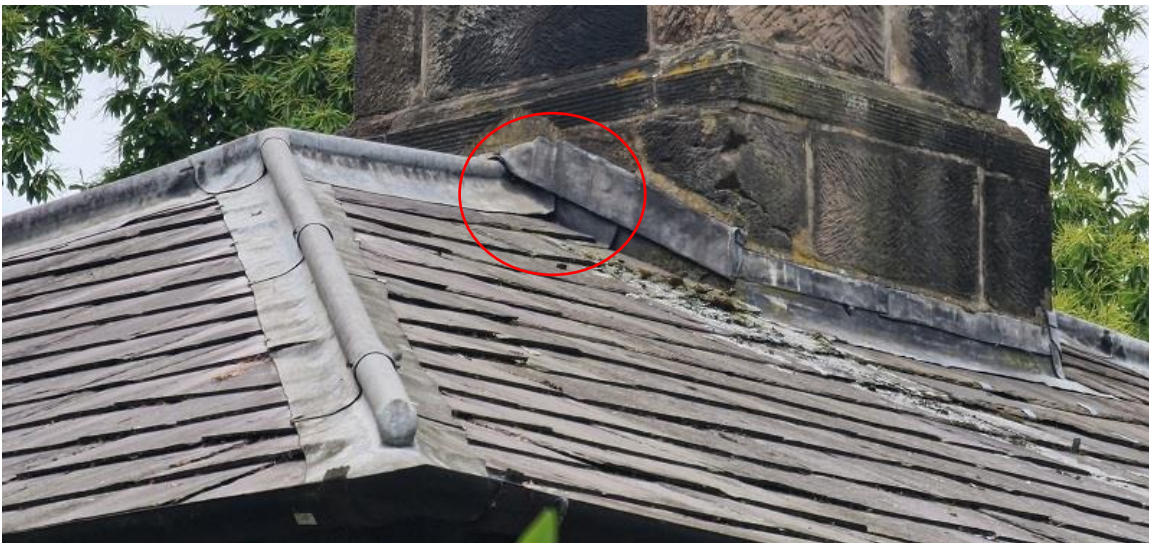
4. Main access point for bats below the ridge, to southeast of chimney
