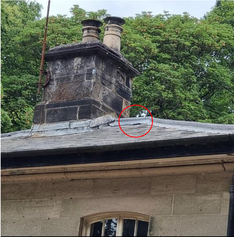
3. One of roost access points – southwest of building
