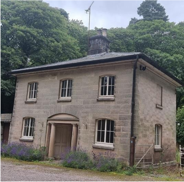
1. North Lodge – southern and western elevations
