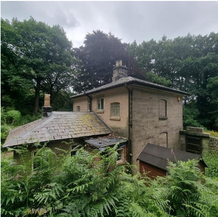
2. North Lodge – northern and eastern elevations including rear extension
