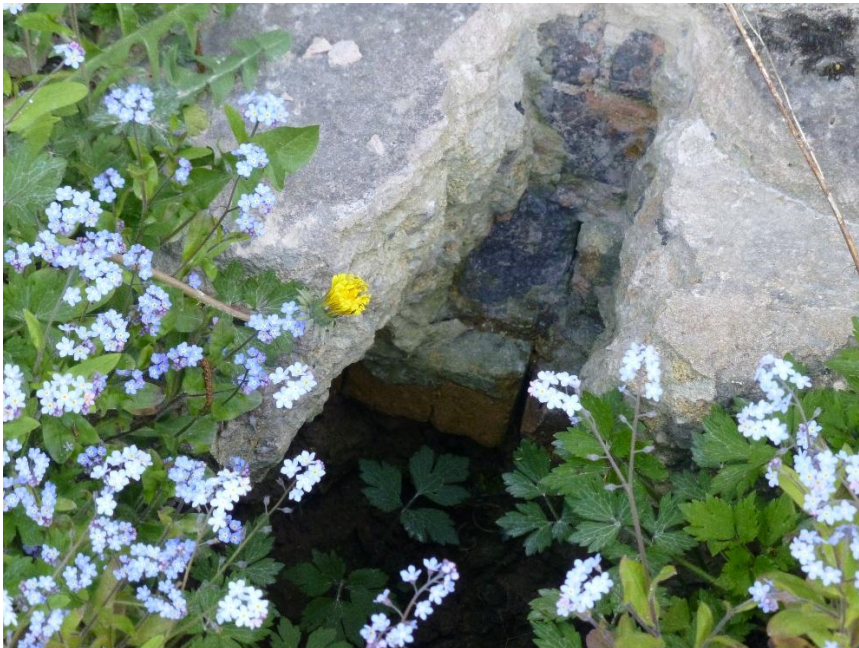
Fig. 6 Existing below ground brickwork
