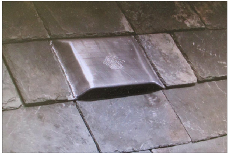
Fig:6 Leadworx – Lead Bat access tile.
