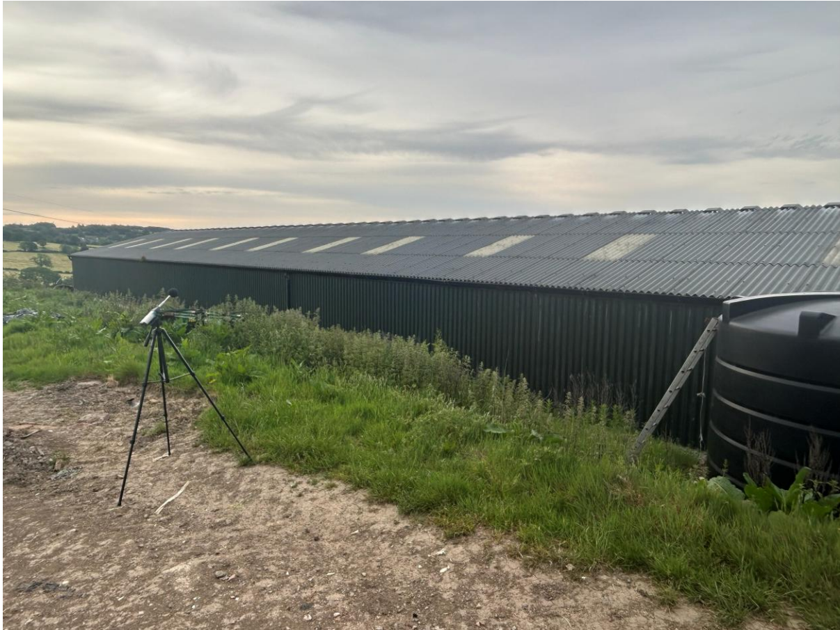
Figure 2: Measurement Location 8m from Building
