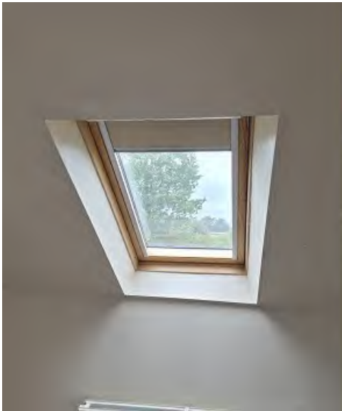
WSW view left dormer bedroom window
