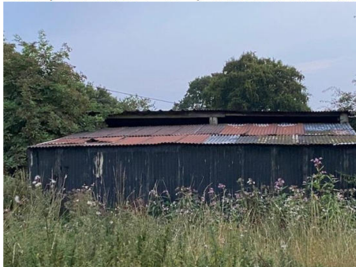
Survey 1 - Position 1 – B7 - (Grid Ref: SK 01696 41050)
