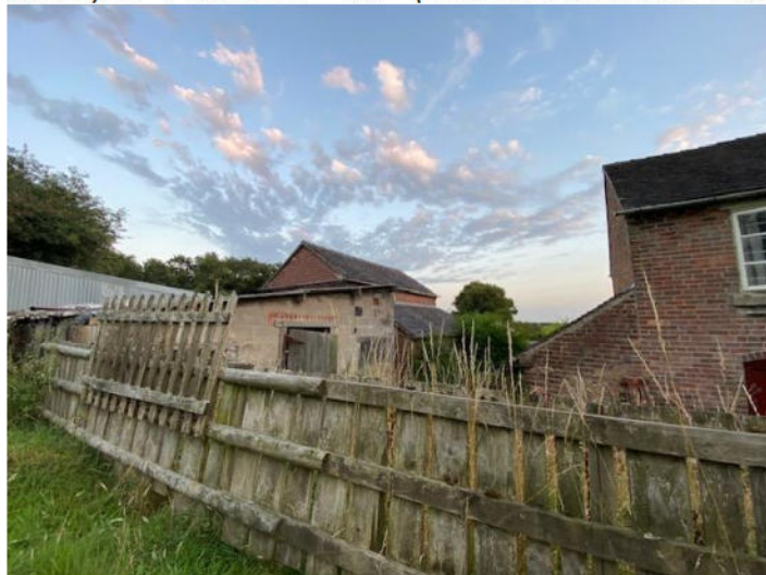
Survey 2 – Position 2 – B3 – (Grid Ref: SK 01667 41048)
