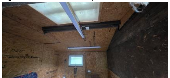
Figure 12. Internal compartment on west elevation.
