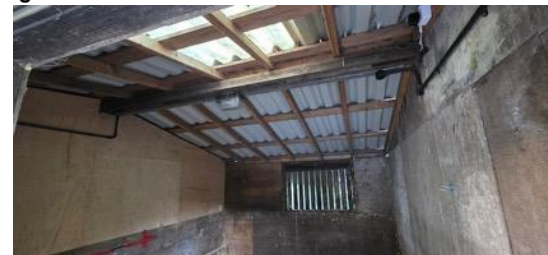
Figure 11. Internal compartment on East elevation.
