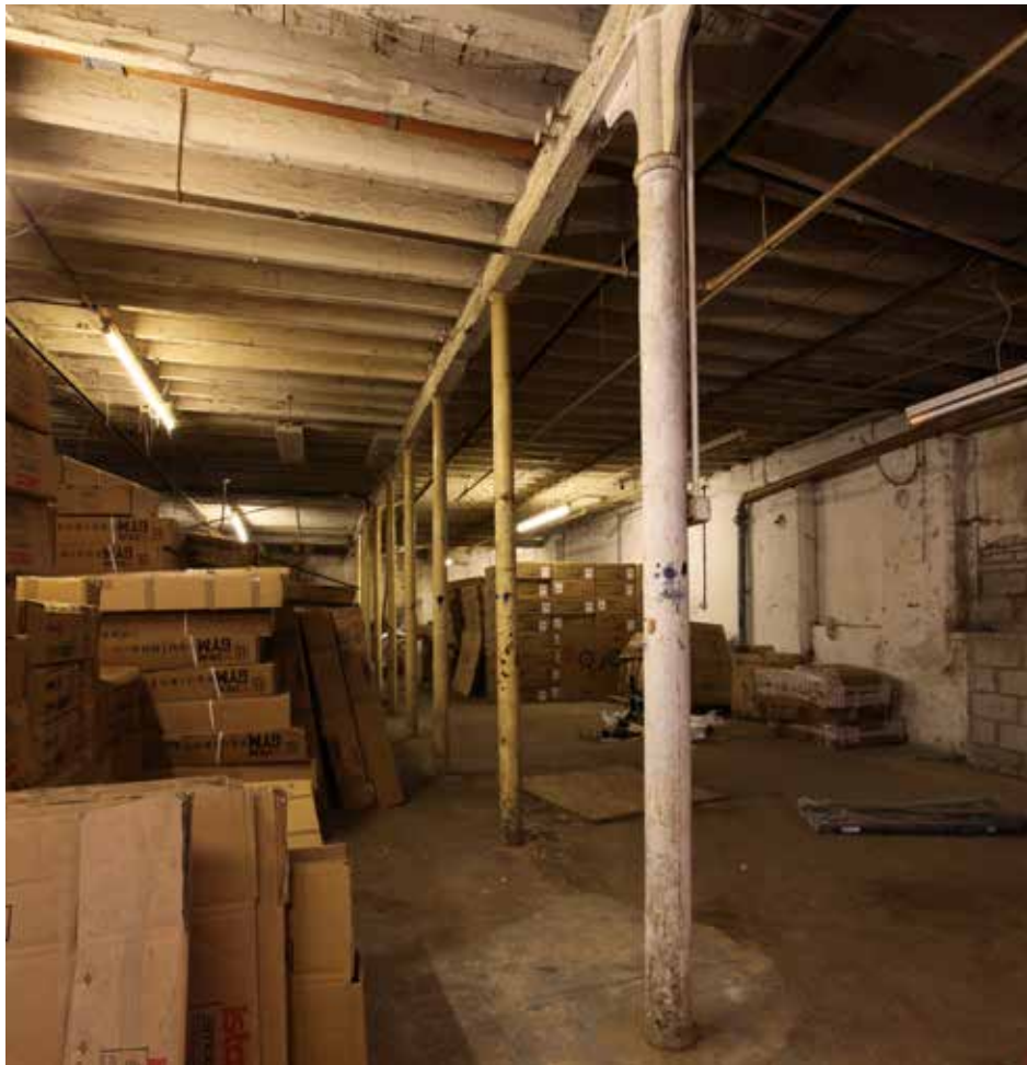
8. Ground floor - cast-iron columns looking west
