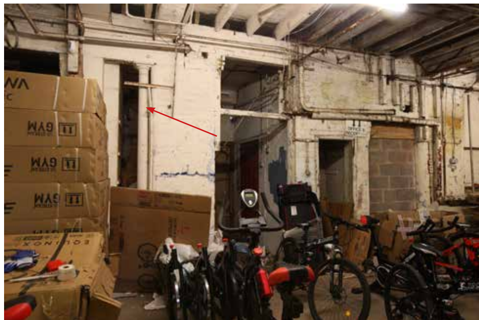
14. The north transept is partially infilled at ground floor level. The cast-iron column (arrowed) may have been added when the transverse beams were inserted, as it appears to be providing additional support to the load from the beam above.
