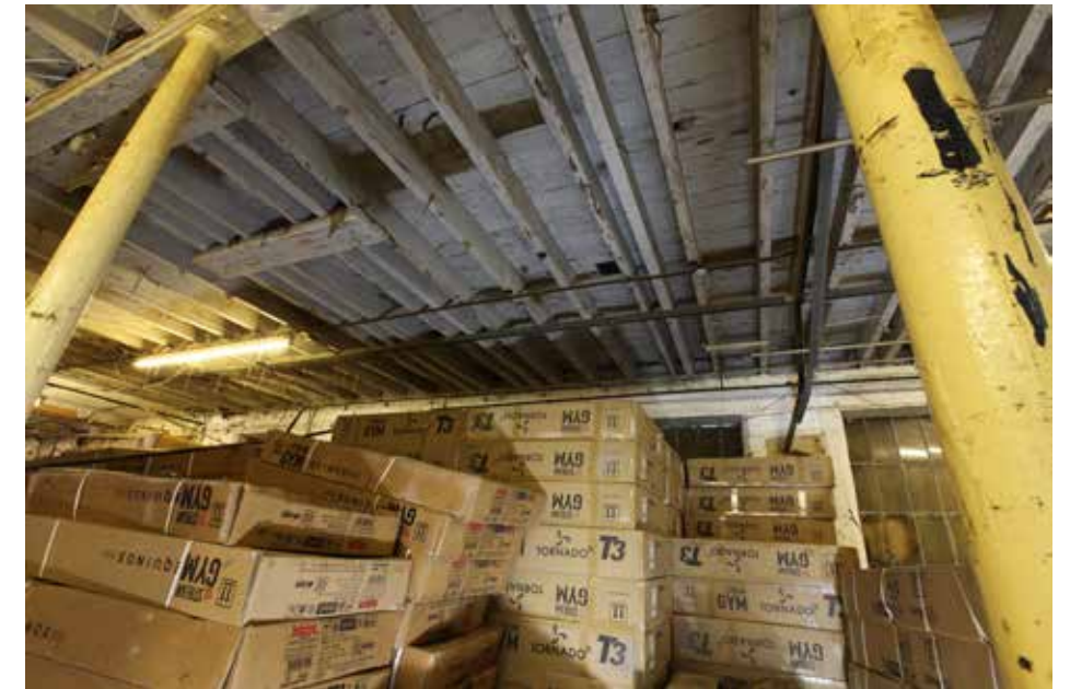
11. Section of ground floor ceiling with supplementary timber joists.
