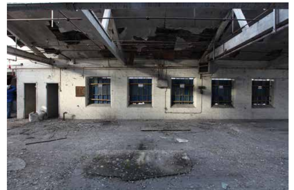
24. Surviving cast-iron windows to rear elevation
