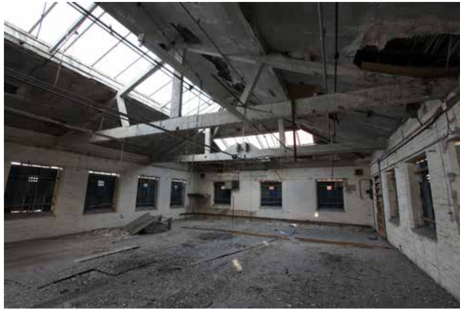
20. Northlights and King post trusses
