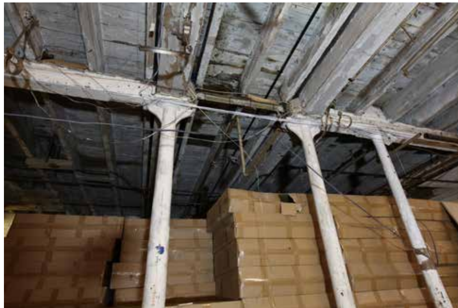
10. Pitch pine transverse beams with replacement flanged cast-iron columns to ground floor ceiling.
