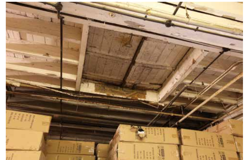
12. Trap doors to former internal hoist.
