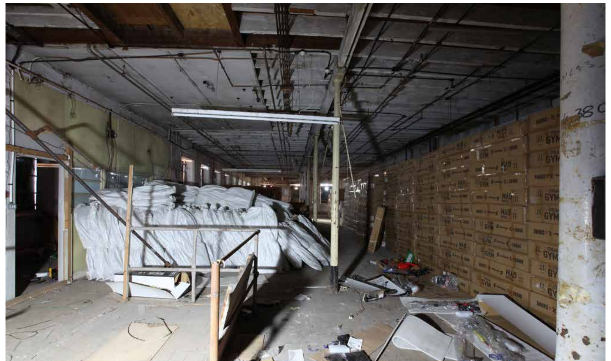
15. Below - first floor with 12 feet floor-to-ceiling height and slender cast-iron columns
