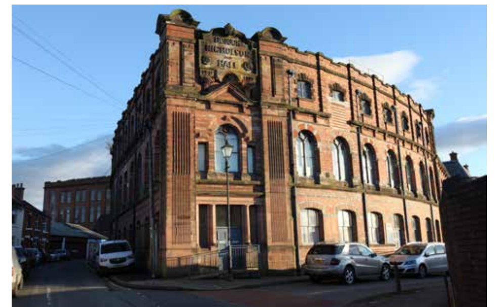
26. Cross Street Mill, with York Mill in the background, are both part of the setting of London Mill.
