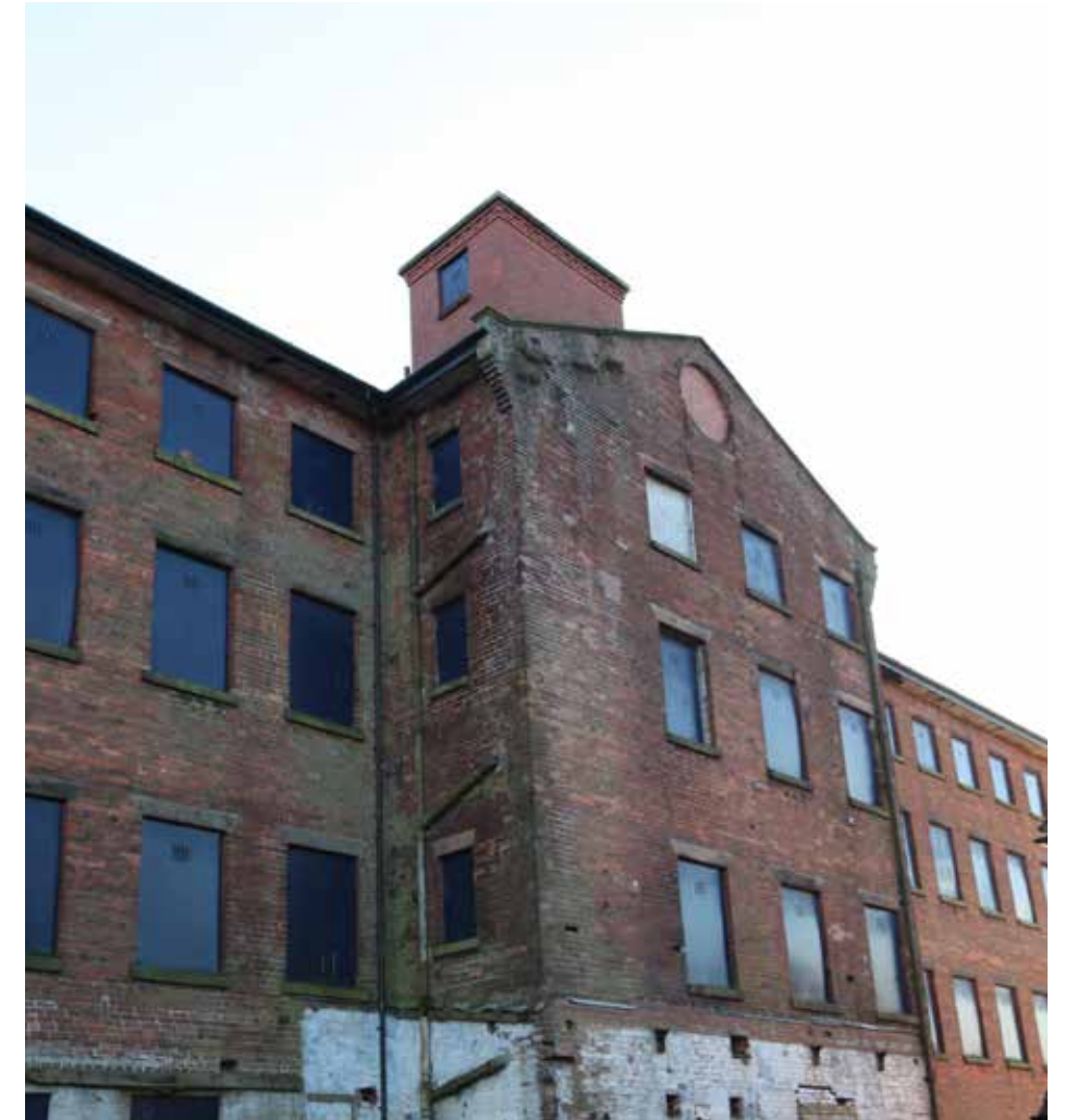
7. Rear transept with former clock face (bricked up) and smaller windows for water closets. Lower down the elevation is the painted face of the former internal wall to the engine room. The modern brick, goods lift over-run is relatively modern (post 1934).
