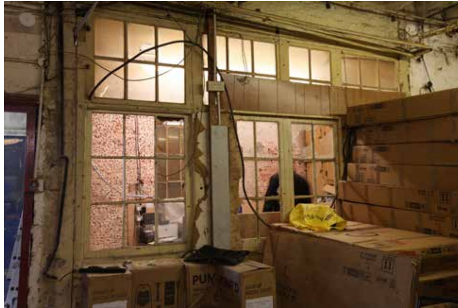
9. Internal screen at ground floor level - this has been modified but may be the remnants of the Counting House.
