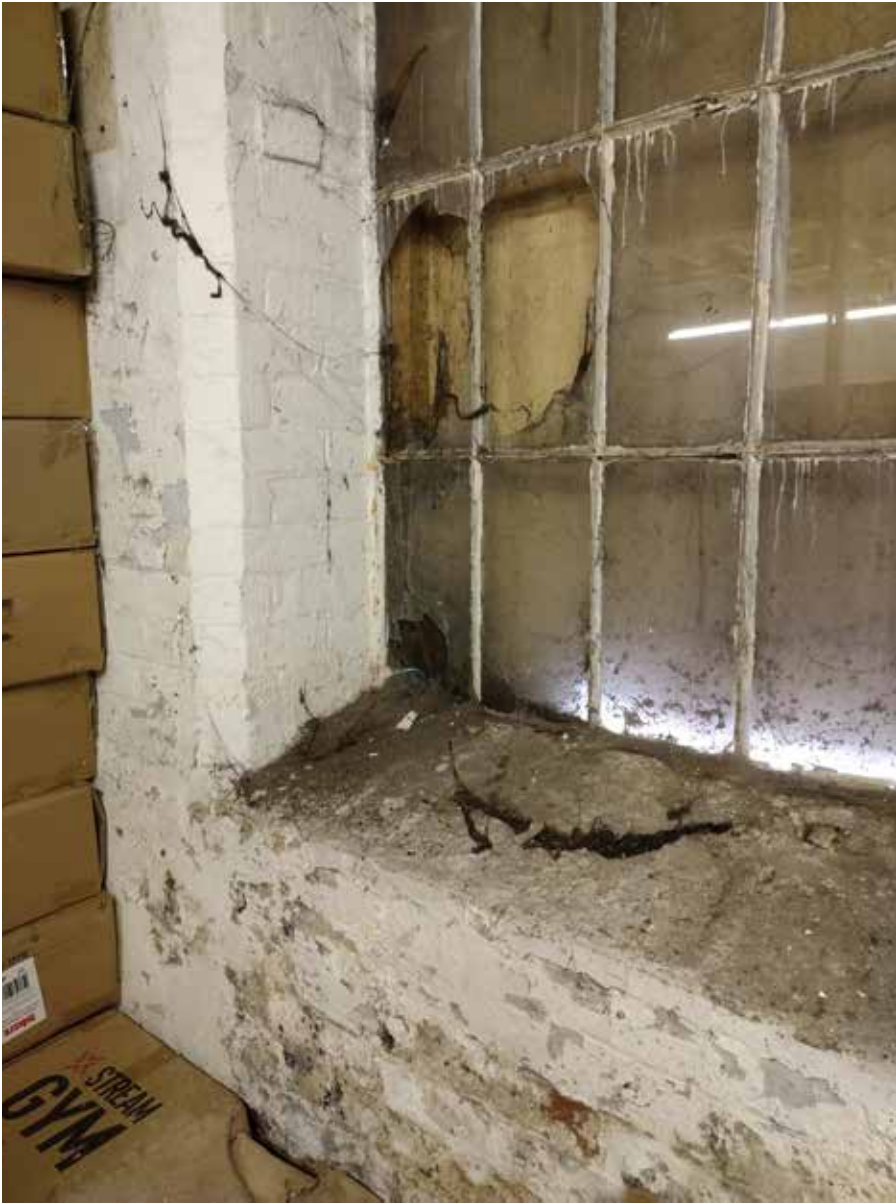
30. Detail of cast-iron window with very fine section glazing bars, putty finish, and 3-4mm glass. Windows were actually glazed internally so that it was easier to replace broken panes.
