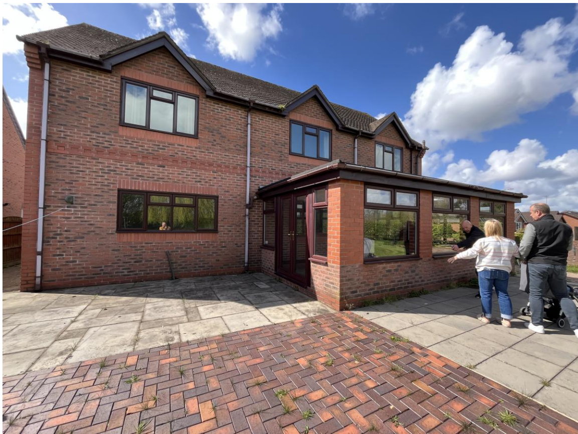
Existing Site Photo
