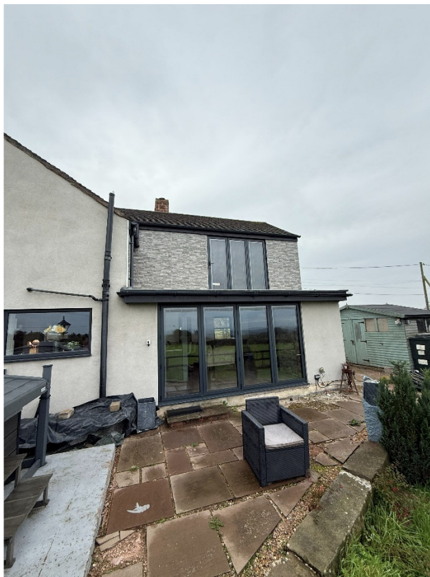
Image 3 – Rear elevation showing former extension & area of works.
