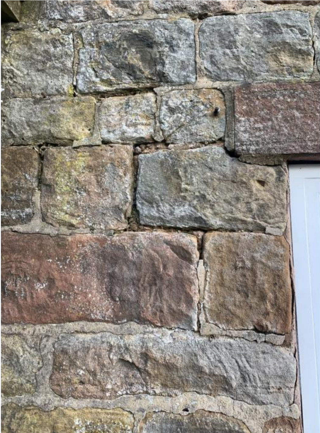
Close Up of the Panel on the South West Elevation
