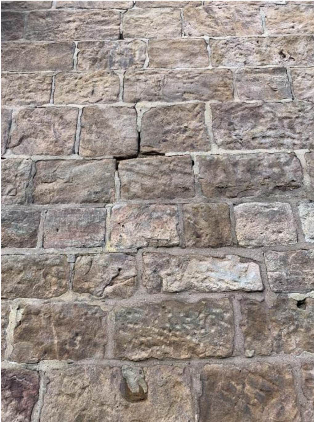
Close Up of the South East Gable End Elevation
