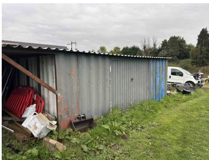
Figure 4: Existing storage arrangement for maintenance equipment and vehicles
