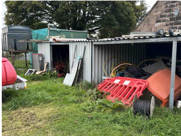
Figure 8: Existing storage arrangement for maintenance equipment and vehicles
