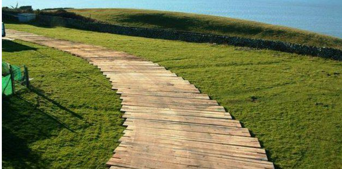
Figure ii- Temporary road example
