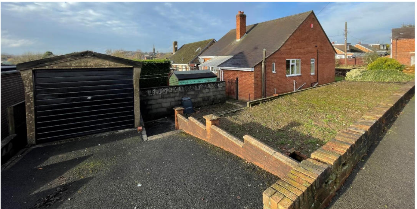
Figure 1: The application site from the Southeast corner where the existing access is from Thorley Drive.
