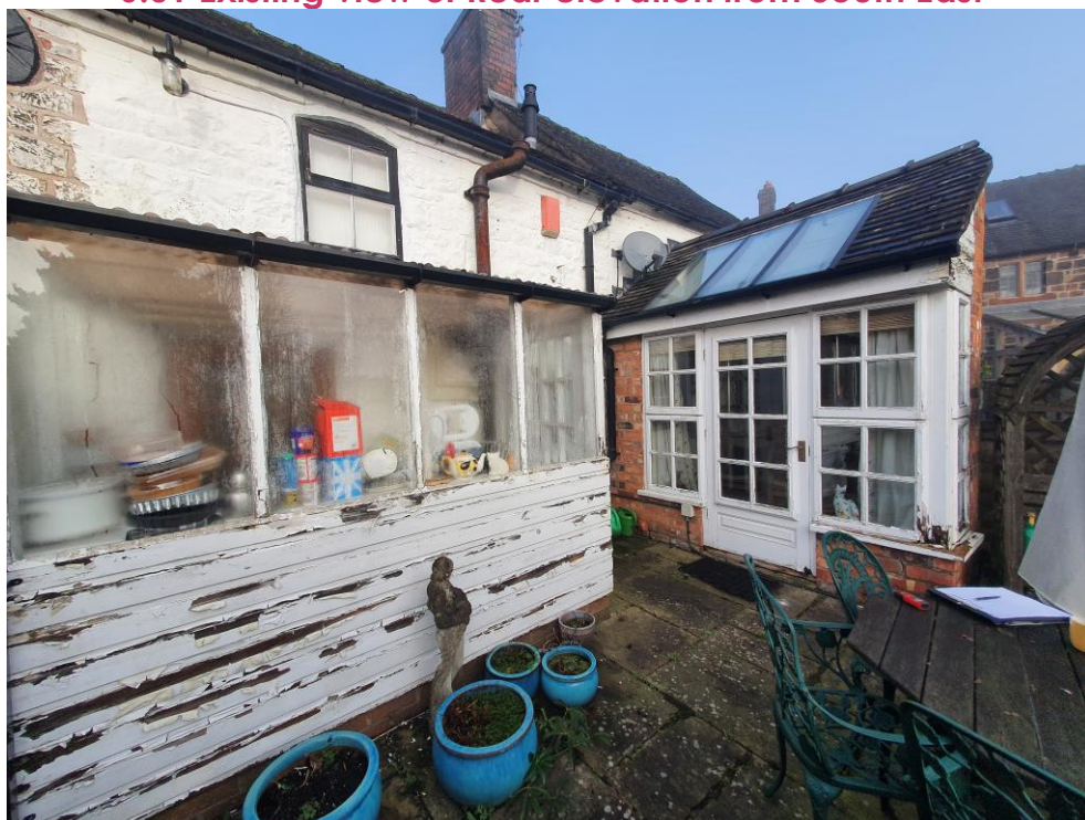
6.01 Existing view of Rear elevation from South East
