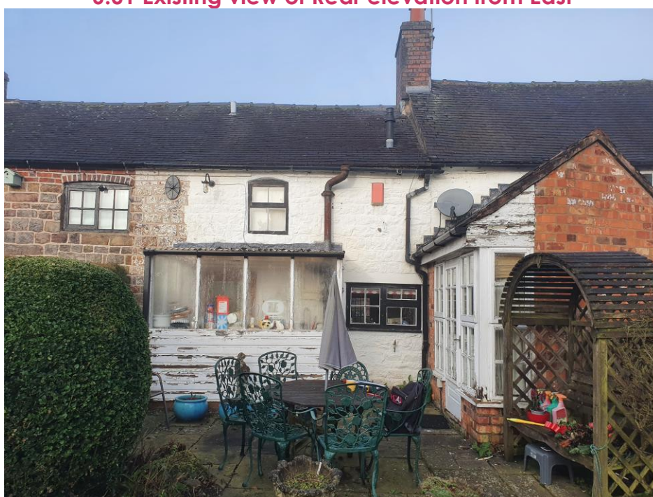
6.01 Existing view of Rear elevation from East
