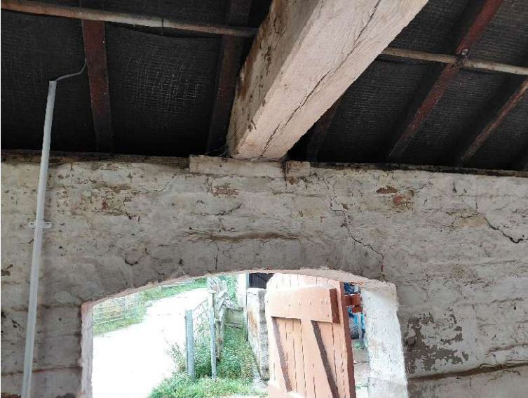
Truss support over doorway
