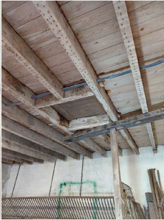
Repurposed first floor with props
