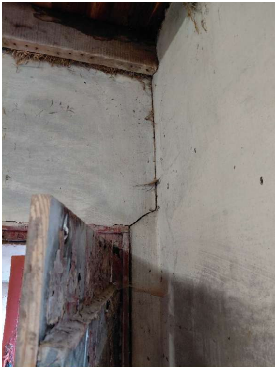
Debonding of buttress walls
