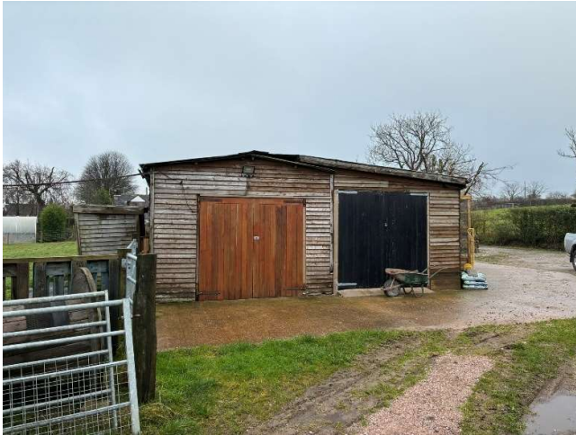
Shed to be replaced
