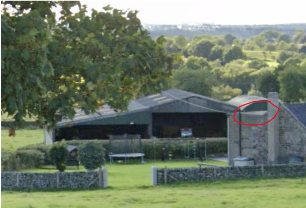
Agricultural building on Park Lane with flat roof extension and timber cladding
