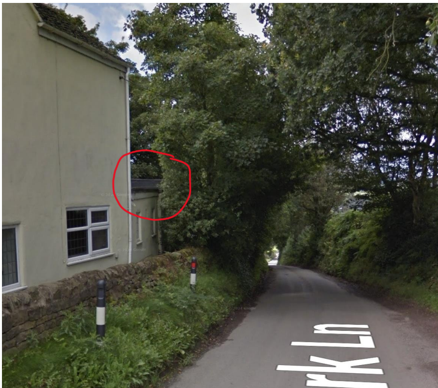
Adjacent property with flat roof extension
