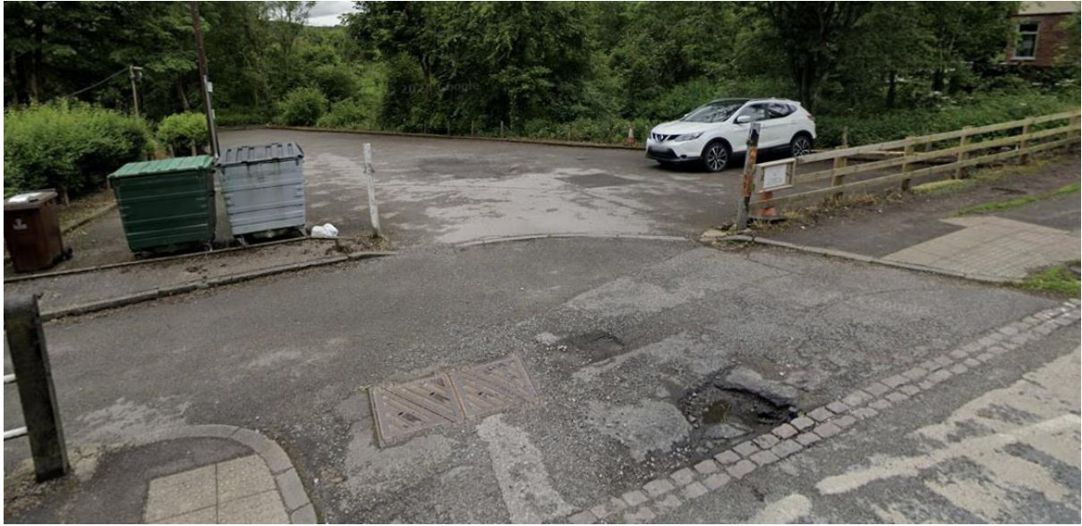
Photo showing access from car park on to small private road then on to Cheadle Road
