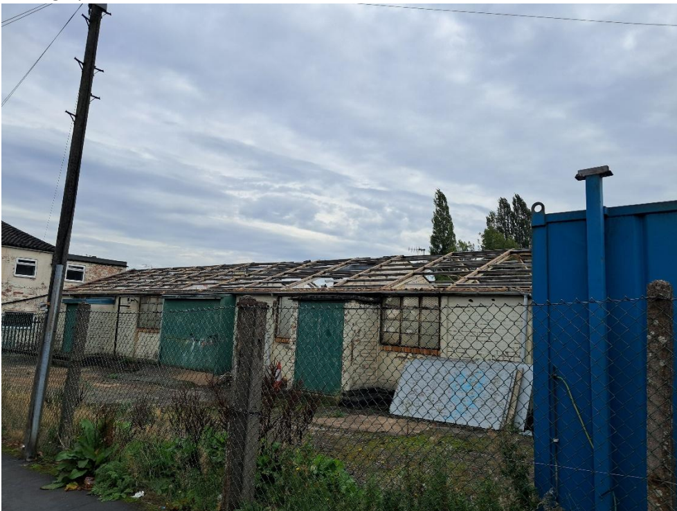
Photograph 2: General view of site
