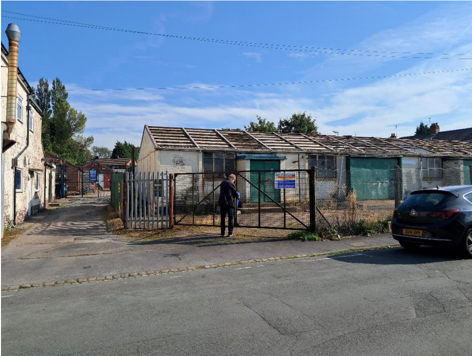
Photograph 1: General view of site
