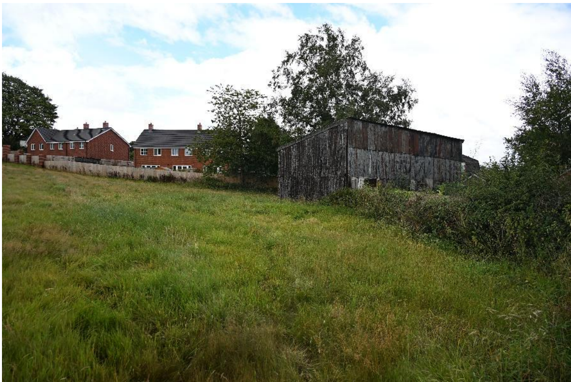
Image 2 South across site to Target Building 1
