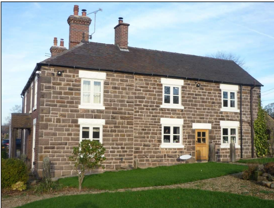
Fig. 3 – south elevation November 2025
