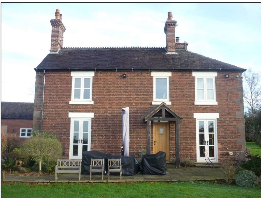
Fig.2 – brick and stone quoin double fronted west elevation
