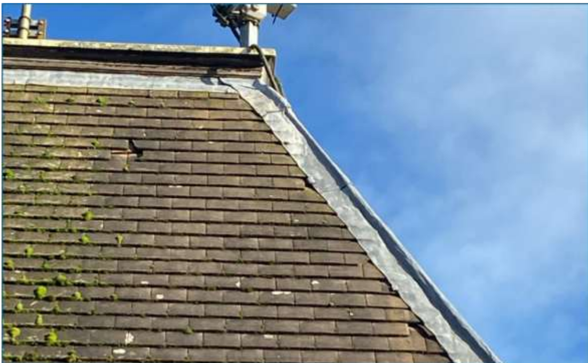
Figure 2. Close up of bat roost feature
