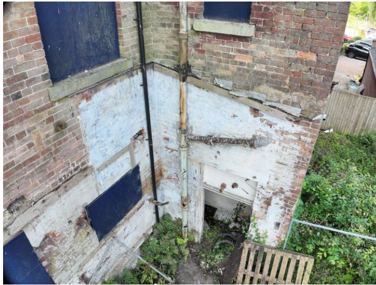
Image 3: Internal painted coatings exposed by demolitions.
