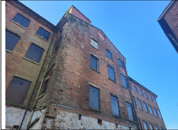
Image 1: North facing aspect, rear of the building.
