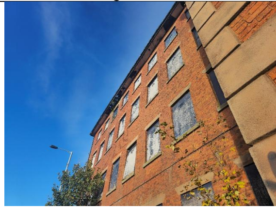
Image 4: South aspect, towards the western aspect of the front of the building.
