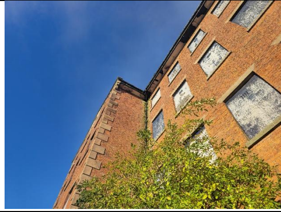
Image 2: South aspect, towards the centre of building.
