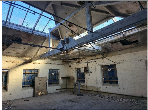
Image 8: Top floor, internal view looking east.
