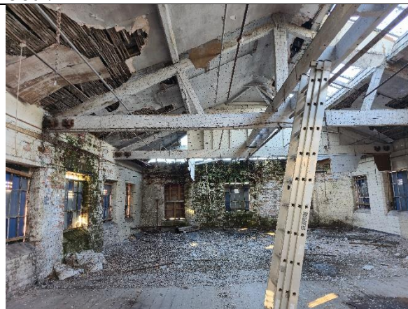
Image 10: Top floor, internal view looking west.
