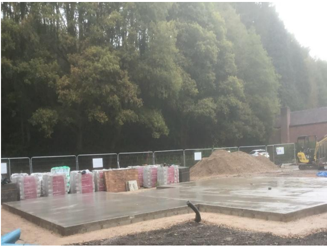
Image 3; Completed raft foundation
