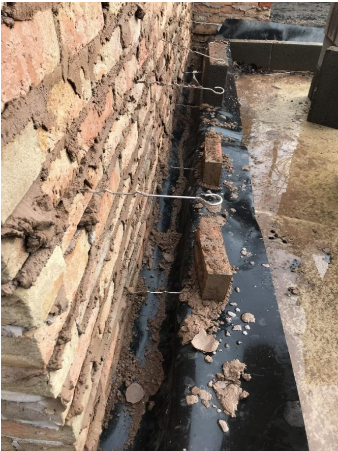
Image 4; Installation of Corden EPS GR DPC
