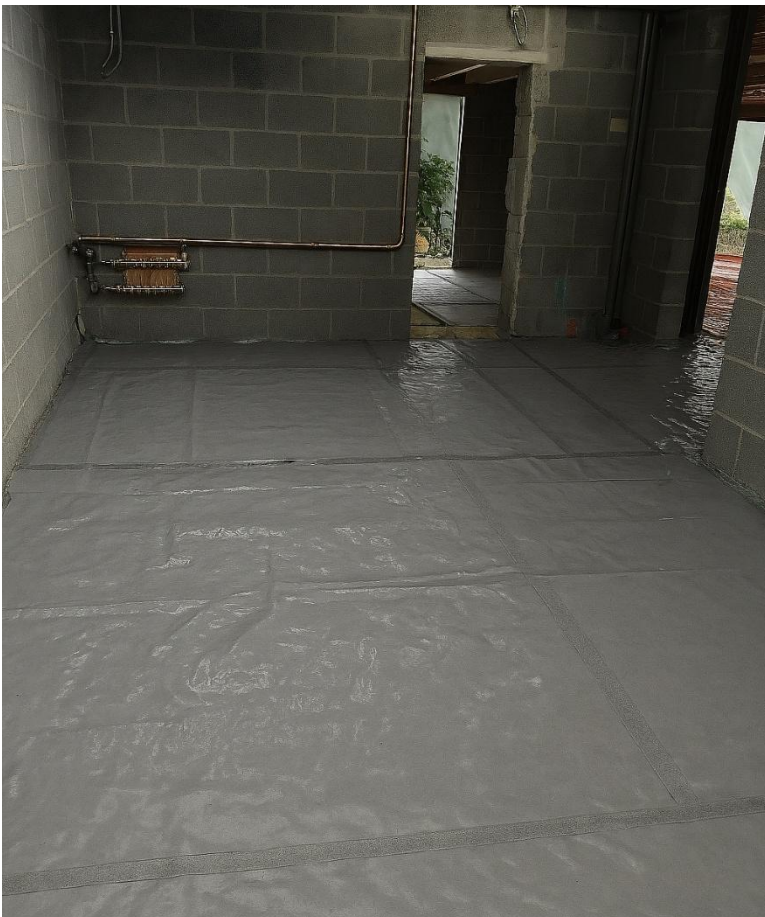
Image 6; Installation of Corden EPS 2000 Gas Membrane fully lapped and sealed using Corden EPS Gas Tape and Corden EPS Lap Tape
