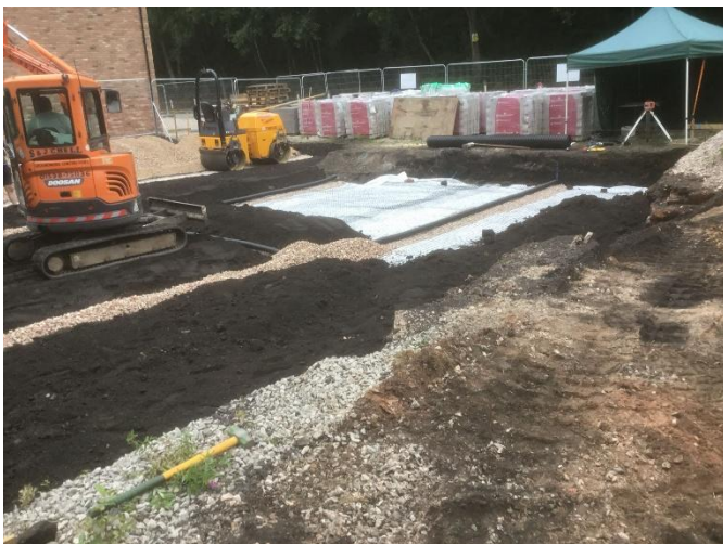
Image 1; Installation of raft foundation inclusive of ventilation run
