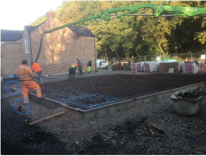
Image 2; Concrete Pour for raft installation, highlighting foundation ventilation.
