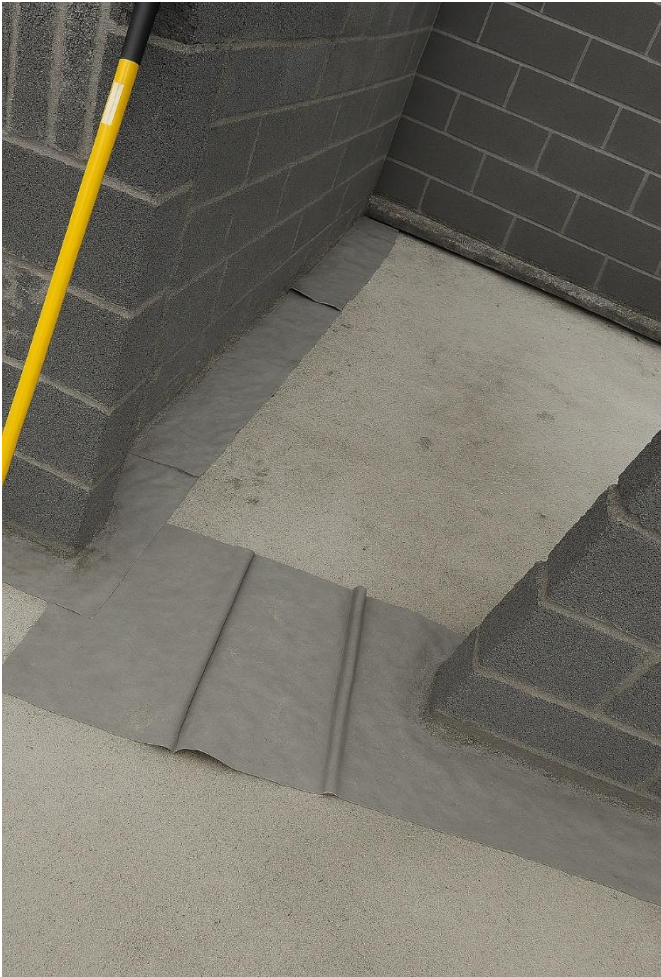
Image 5; Installation of Corden EPS 2000 Gas Membrane below internal wall structures and lapped to the underside of EPS GR DPC
