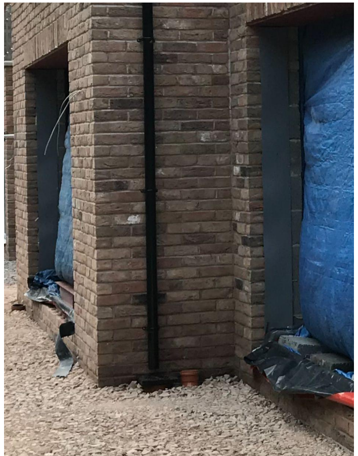
Image 8 & 9; Showing Foundation ventilation ducts as per specification
