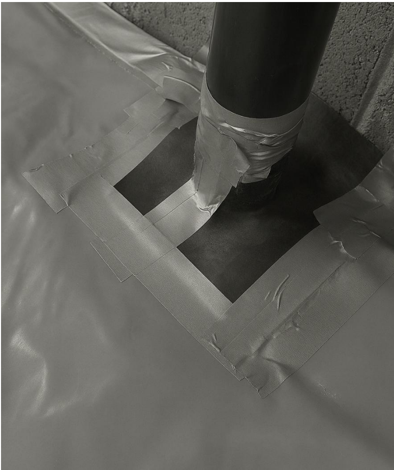
Image 7; Showing installation of Corden EPS Preformed Pipe Collars
