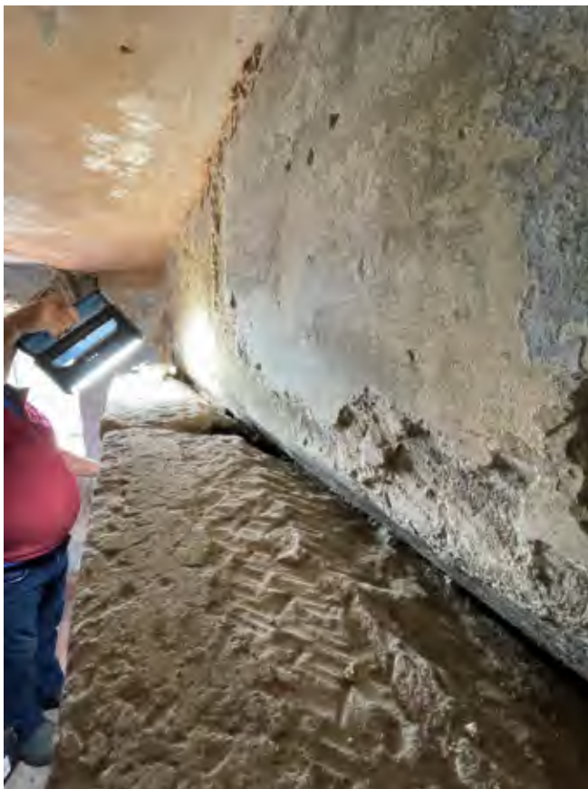
13. Corner fireplace with stone masonry chamfered surround to the full-height of the ceiling of ca. 1680 in-situ. This detail shows the chamfer intact with the back of the later stone surround tooled to avoid defacing the original chamfer. This was filled in a weak mortar and the face of the hearth of 1680 was given a thin coat of lime plaster, which has become largely detached.
