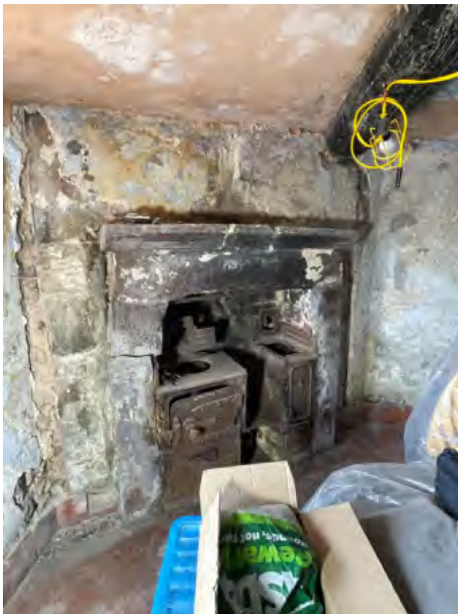
11. Corner fireplace to Parlour in southern bay of ca. 1680., with two phases of stone surround and cast-iron range of the 19 th century. Lath-and-plaster ceiling, with gypsum skim in places.
