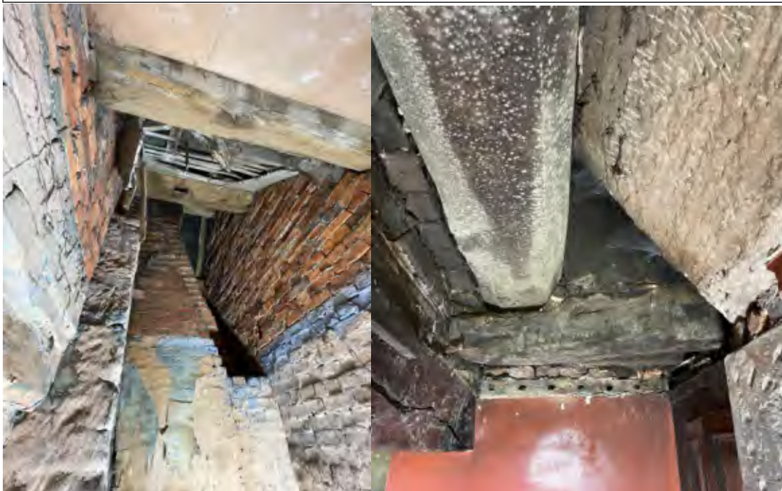
21. Left – inserted brick chimney breast (mid C18) & 22. Right – inserted sloping slab and lintel (ca. 1743).
