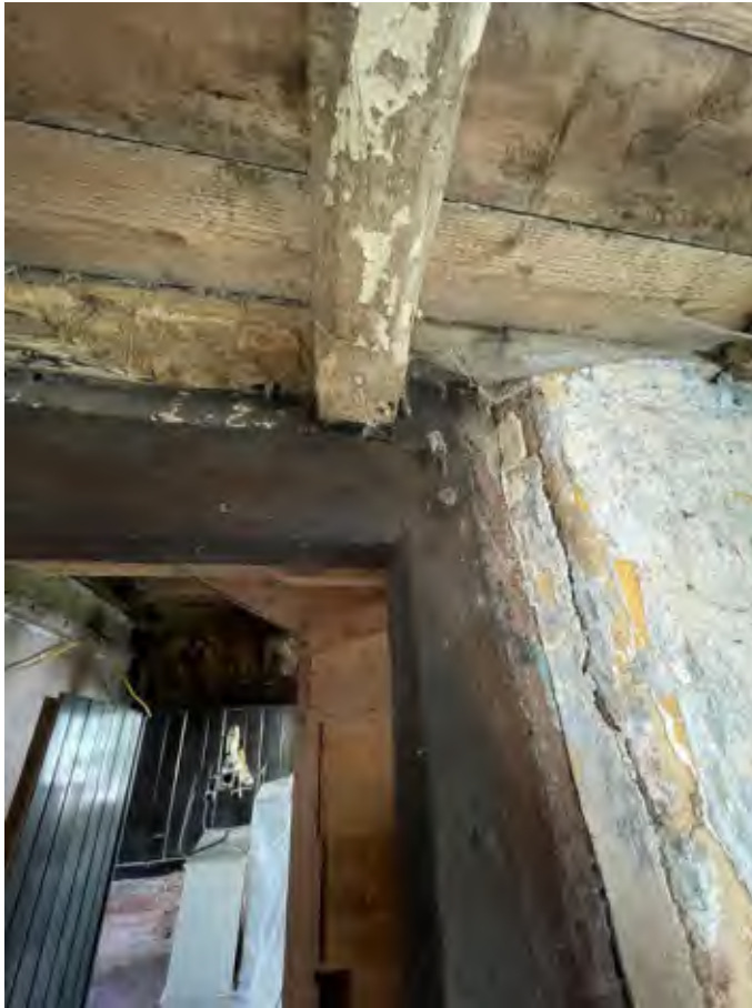
16. Pegged oak door frame of 1624 with inner door reveal to lobby inside main entrance. Stop-chamfered oak joist and later boarded floor.
