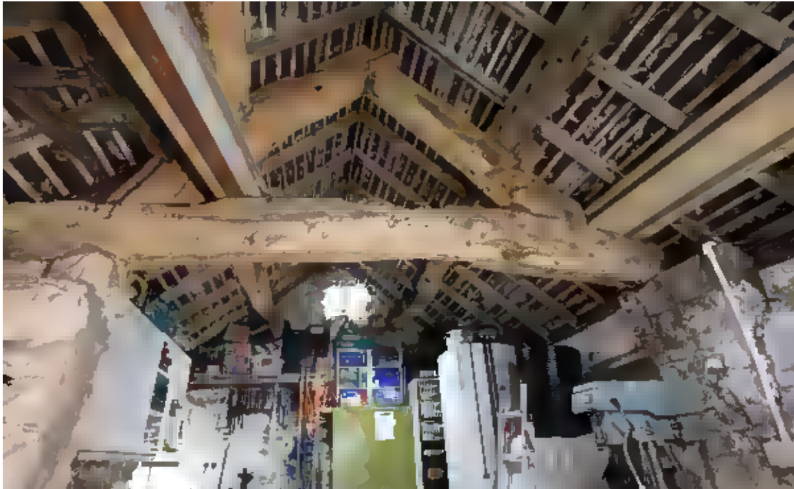
38. 17 th century truss inserted into centre of stable roof over cross wall, which has been part demolished.
