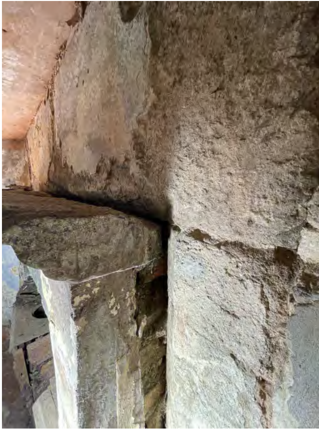
12. Corner fireplace with stone masonry chamfered surround to the full-height of the ceiling of ca. 1680 in-situ, and later inserted stone fireplace of the early 19 th century with moulded lintel.
