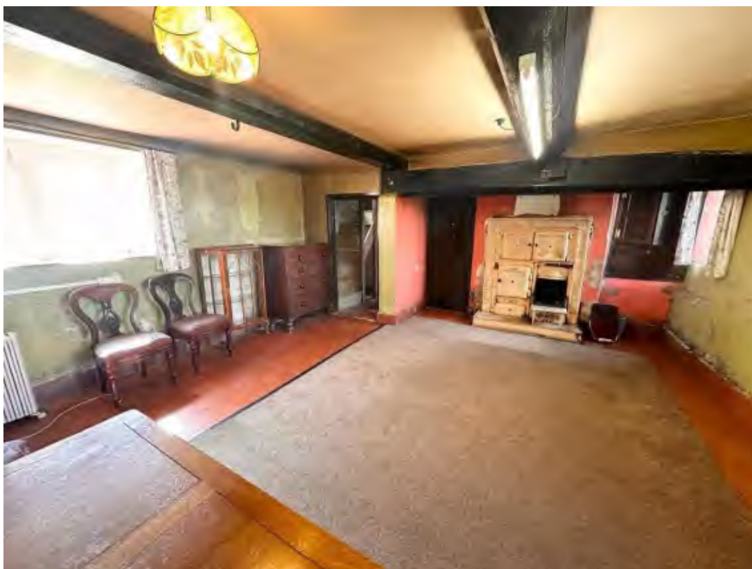
18. View of the interior of the Living Room from the sale particulars. Ceilings are plasterboard and have been removed to inspect the condition of the oak joists.
