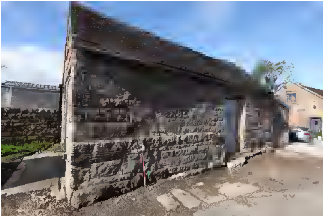
36. Stable – 17 th century form with deep plinth and large blocks of masonry, altered and extended at the end of the 19 th century.
