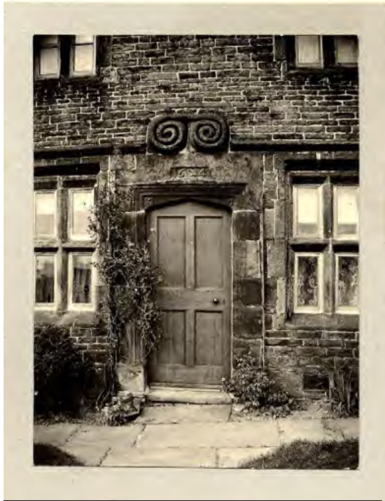
Fig. 9 Example of a building of 1624 in South Yorkshire with full double-chamfered stone window surrounds and similar shaped door lintel.
