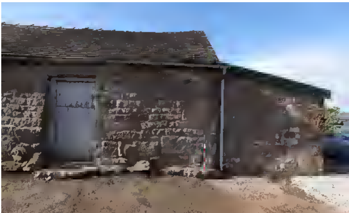
37. Stable – 17 th century with later alterations and large blocks of masonry. Lean-to addition of the late 19 th century in stone.
