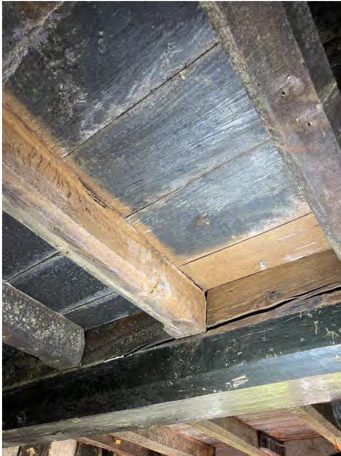
32. Main Living Room – area of test steam cleaning to soffit where plasterboard has been removed and revealed stop-chamfered oak joists and boarded ceiling.
