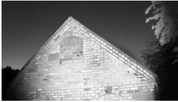
Image 7: infrared still image of southern gable wall taken at the darkest part of the survey on 14th June 2025. Note that views across the easterly roof pitch are somewhat restricted due to the hedgerow (right-hand side of the frame)
