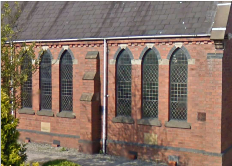
Fig. 2 – close up street view in 2011 of the original windows
