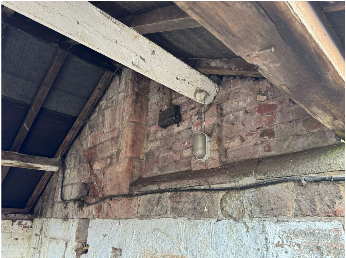
Above & below – stone wall with existing cabling and battery unit location.
