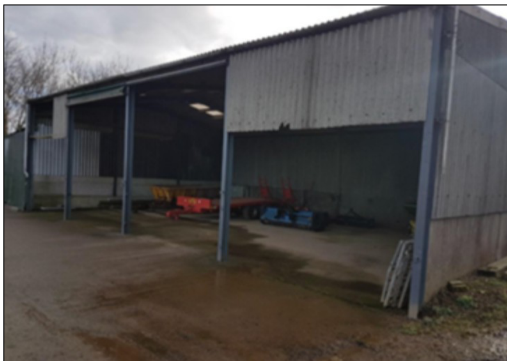
Figure 1 – Image of Building granted prior approval under appeal 3208377
