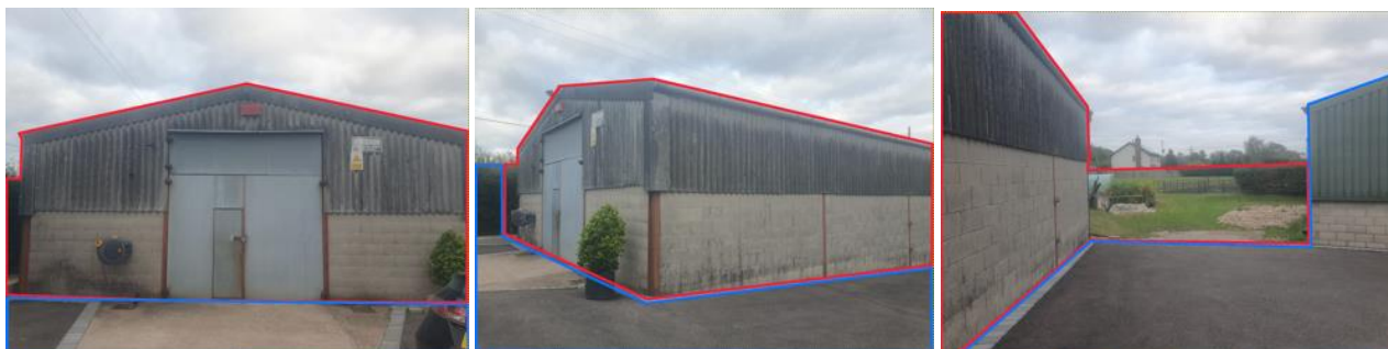
Figure 4, 5 & 6. Agricultural farm building positioned on the North west boundary of the site.
