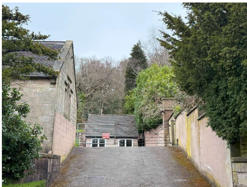
Access to the courtyard with the Annex on the left
