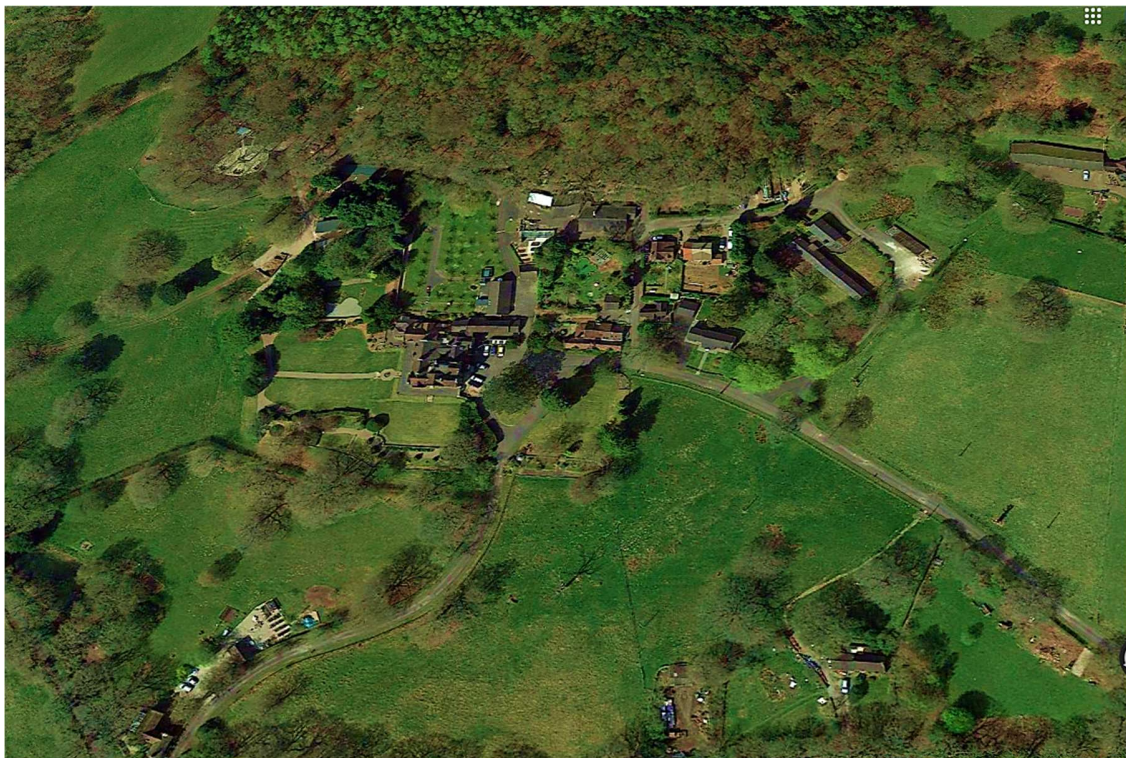
Aerial View Moor Court Hall
