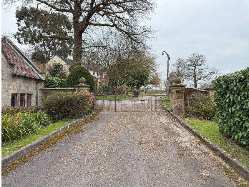
East Entrance – view of Coach House, piers and gates
