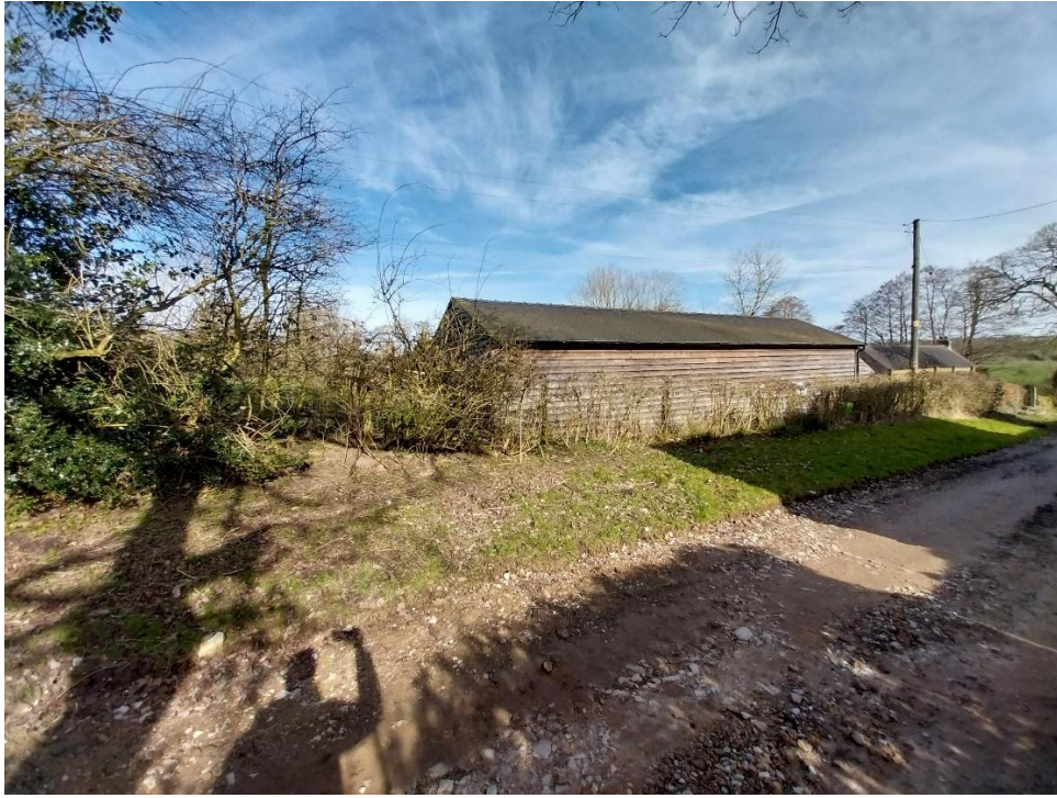
1.View of stables from School Lane.
