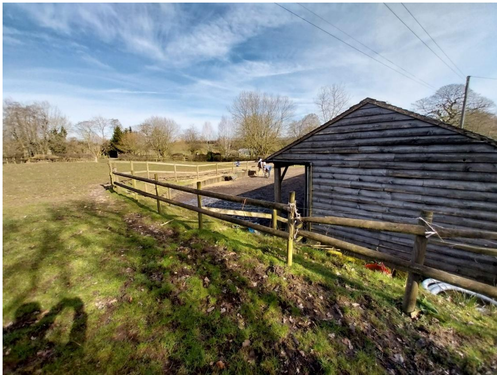
2.West side elevation of site and stables.
