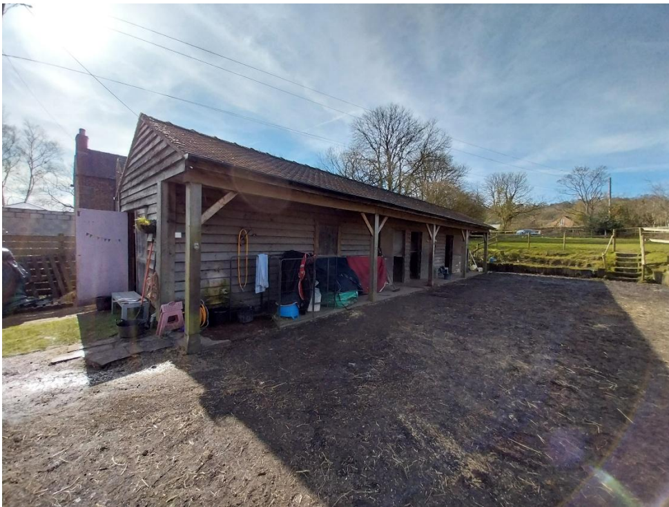
4.Front elevation, east side of stables and yard.
