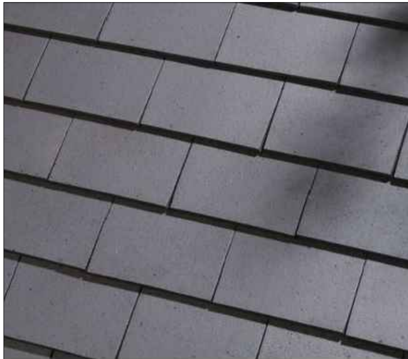
Traditional pain roof (Staffordshire Blue's) tiles to match the existing dwellings in the village.
